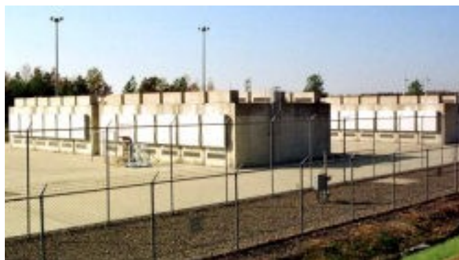
Figure 4. SNF storage in concrete silos in U.S.A.( www.yuccamountain.org )
