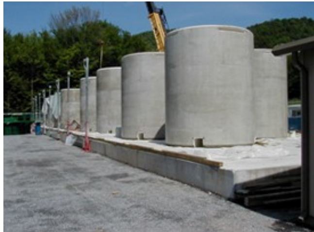
Figure 6. Concrete cask installations (www.nacintl.com)
