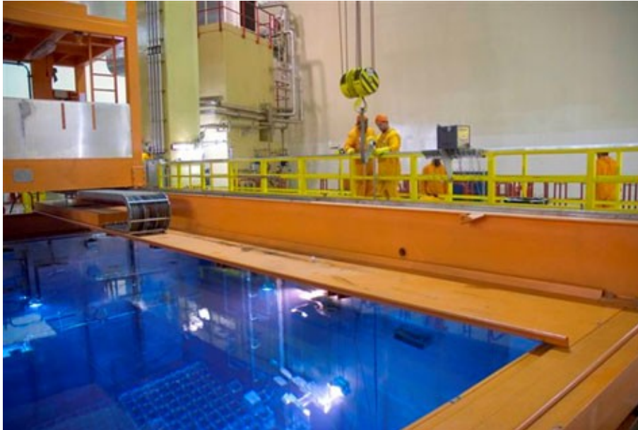
Figure 2. Spent fuel pool (www.eletronuclear.gov.br)
