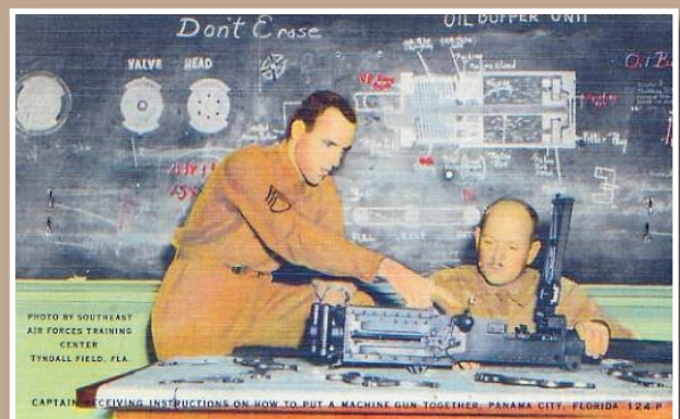
This original color postcard from Tyndall Field, Florida shows a Captain receiving instruction in the reassembly of a .50 caliber machine gun.
