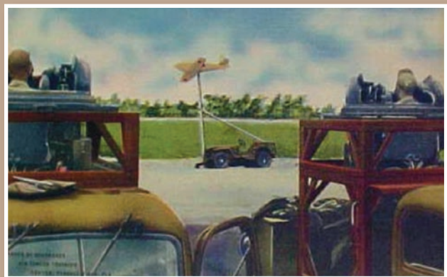
Color postcard from Tyndall Field Gunnery School shows Martin turrets mounted on trucks with an airplane mockup mounted on a jeep. The jeep is hooked to a track system.
