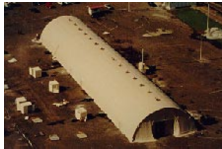
Figure 30. Framed-Support Tensioned Fabric Structure.
