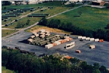
Figure 38. ISO Container Facilities.
