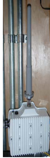
Antenna for data exchange with GE/Silver Springs meter on the other side of the wall
