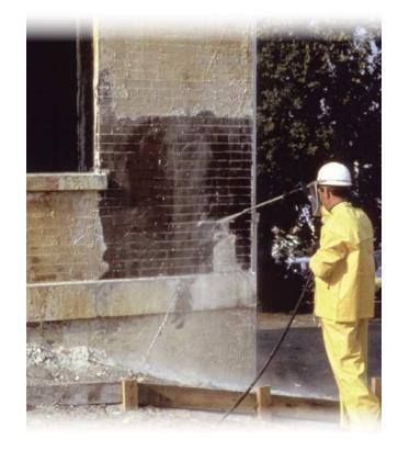
**A worker uses** a simple fresh-water rinse on Knoxville City Hall, Knoxville, Tenn., after paint stripping with Sure Klean® Heavy Duty Paint Stripper. The gel-consistency stripper clings to, loosens and dissolves multiple layers of paint that have been applied over many years. After a sufficient dwell, the spent product and stripped coatings are simply rinsed away.
