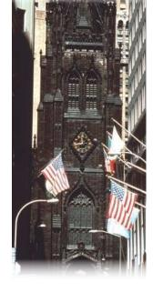
Parts of the spectacular gothic spire on New York's Trinity Church were so decayed, they were too weak to be repaired during the church's restoration. After a thorough cleaning with PROSOCO products, the spire's stonework was strengthened with Conservare® H100 and OH100 Consolidation Treatments.
