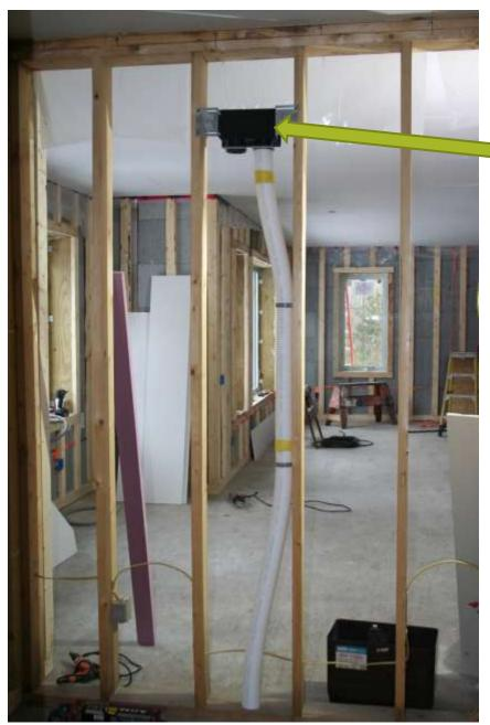
Zehnder Vents to be placed within the Passive House Envelope and not in the ceiling
