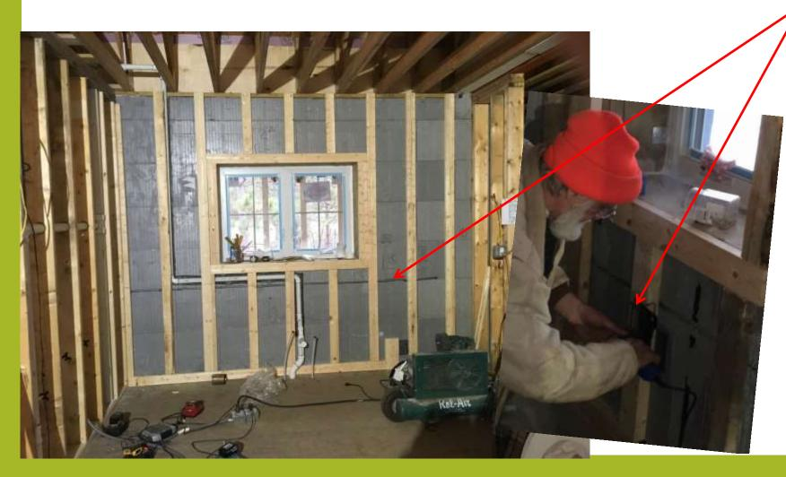
Less room on the main floor to run electrical & plumbing on outside walls. We used a hot knife to cut the ICF foam, installed the electrical & plumbing then foamed over it.
