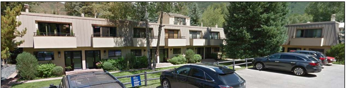
Figure 5: Street View- Looking Northeast from Dean Street
