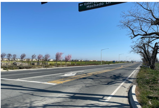
E. Cypress Road Widening (Machado to Sellers)
