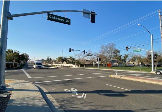
G. Empire Avenue & Gateway Drive Signalized Intersection
