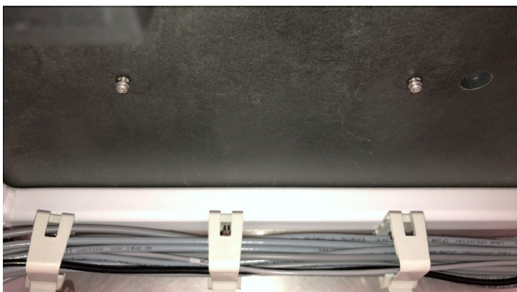
Figure 17 Condensation pump mounting screws partially installed
