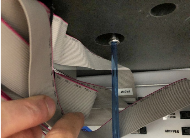
Figure 13 Drainpipe attachment to the cooling unit enclosure
