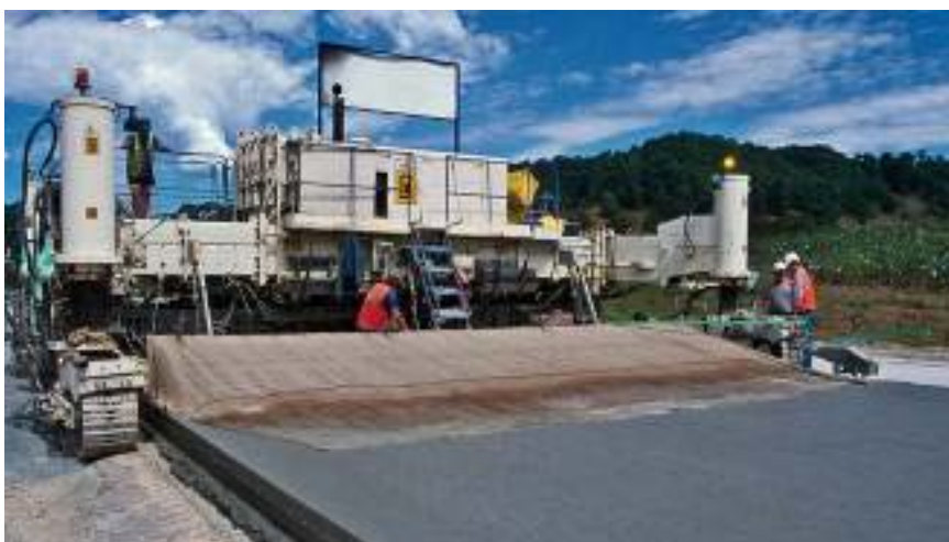
Figure 10.14: Damp hessian being dragged behind a slipform paver
