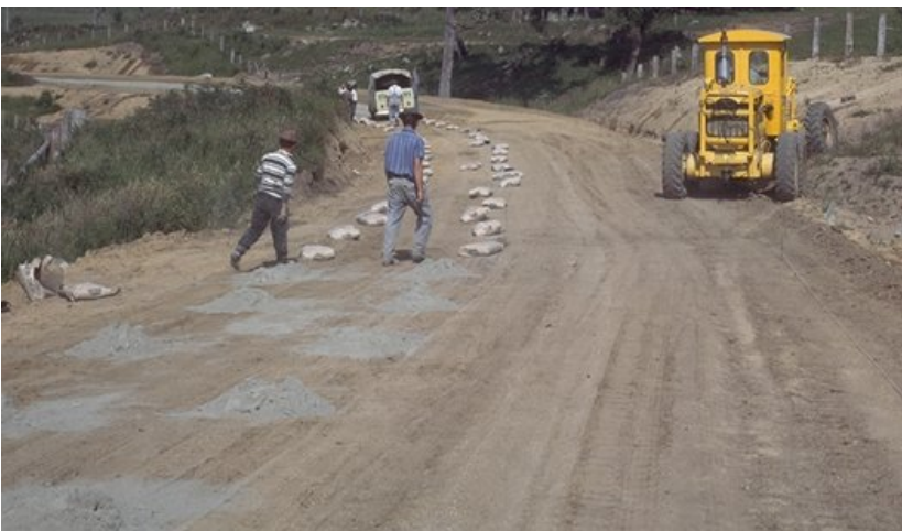
Figure 7.3: Spotting cement bags and hand raking binder into position
