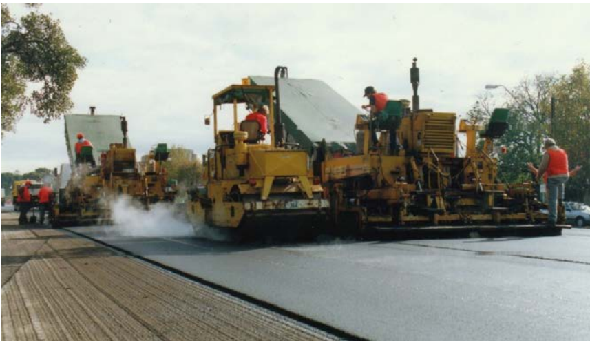
Figure 9.11: Paving in echelon (hot joints)
