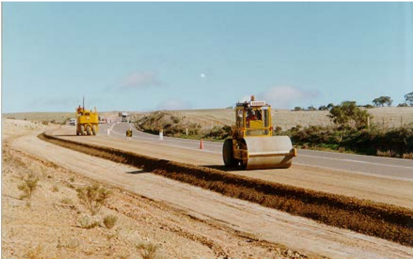
Figure 7.16: Smooth drum and rubber tyred roller in operation
