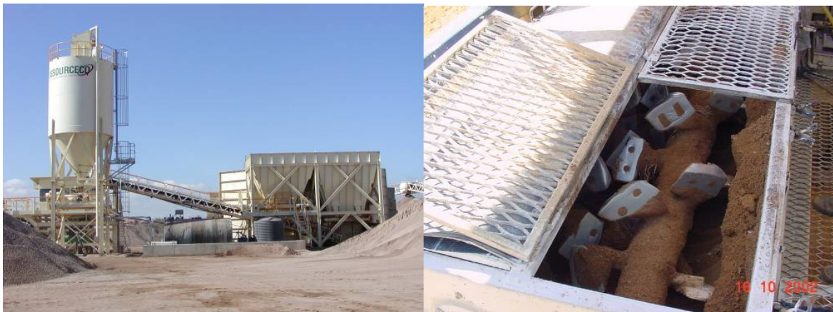
Figure 7.18: Stationary mixing plant and pugmill chamber
