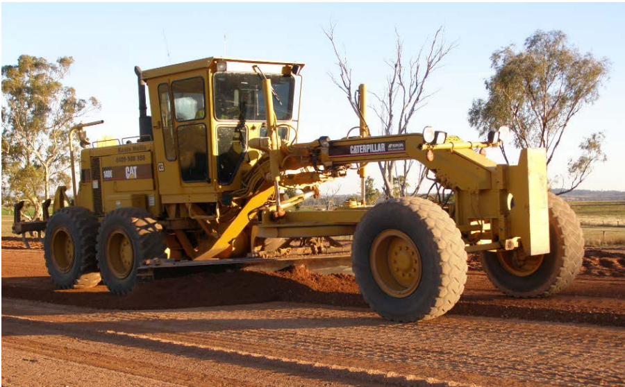
Figure 6.2: Grader trimming granular material
