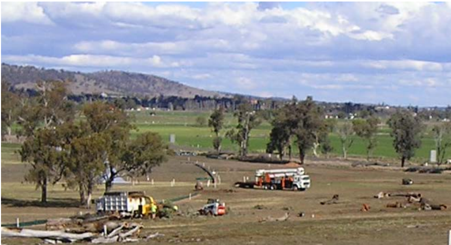
Figure 4.3: Clearing of earthworks alignment
