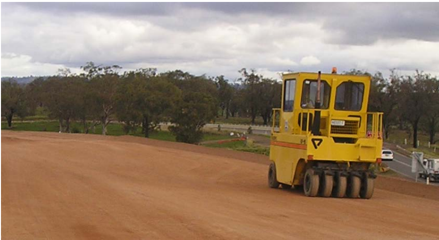
Figure 4.20: Pneumatic multi-tyre roller compacting fill material
