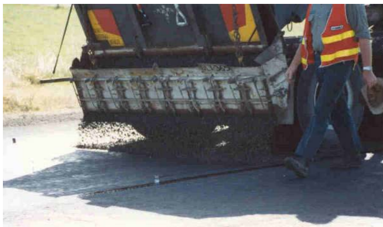
Figure 8.6: Truck mounted box spreader
