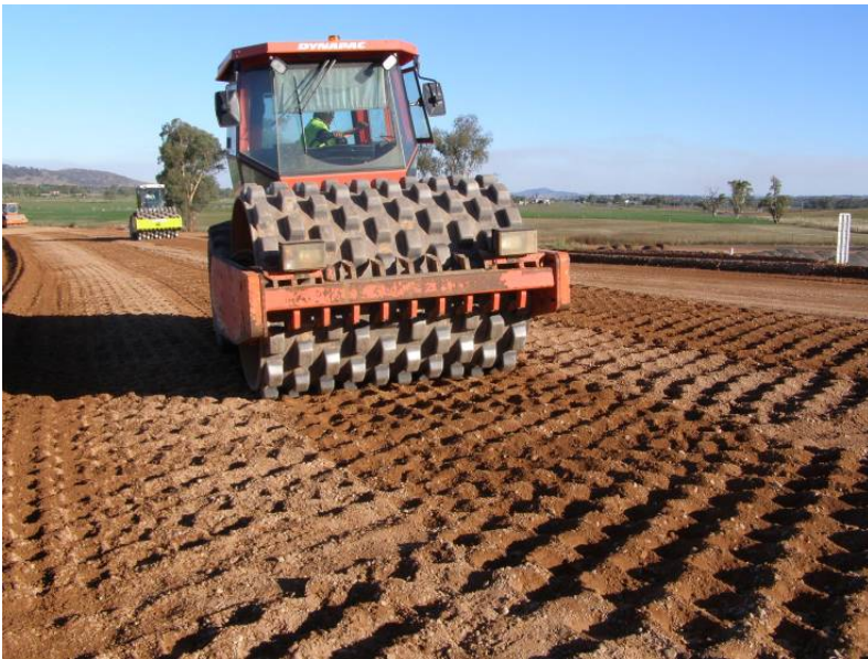
Figure 4.21: Padfoot rollers compacting earthworks fill material
