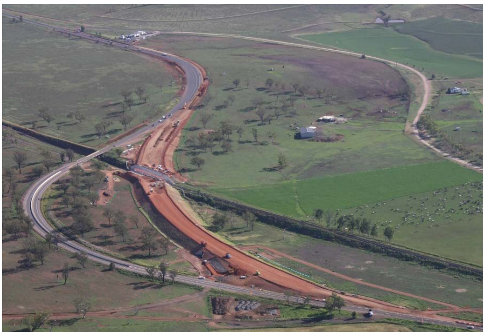
Figure 3.1: Aerial view of a typical rural construction project
