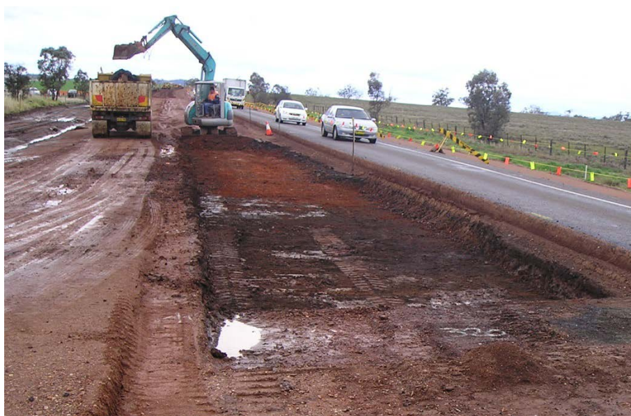
Figure 4.4: Excavation of unsuitable material
