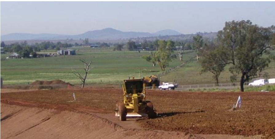
Figure 4.15: Grader spreading earthworks material
