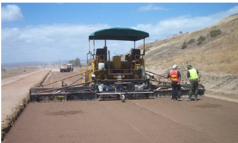
Figure 7.19: Paver laying stabilised material
