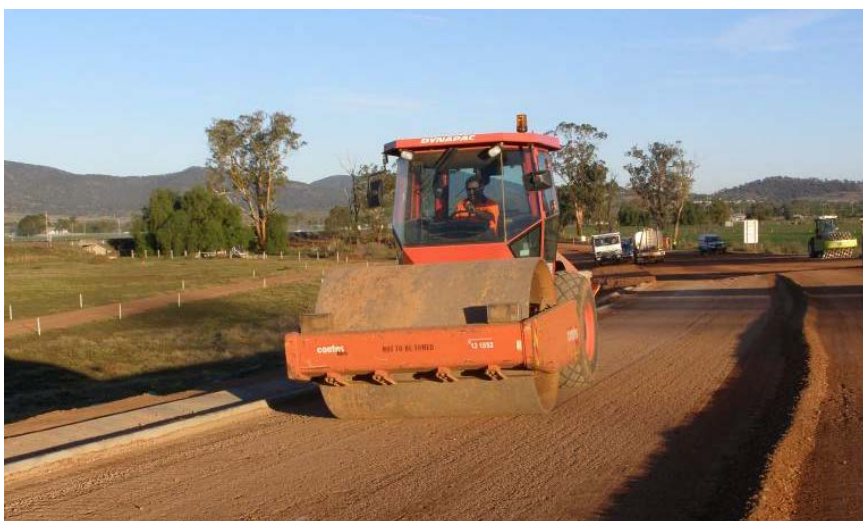
Figure 6.4: Smooth drum steel-wheeled roller compacting granular material
