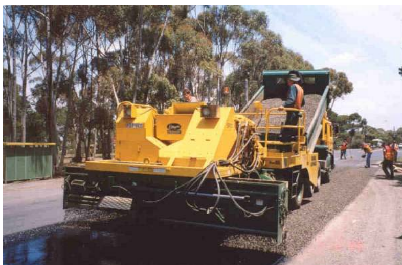
Figure 8.7: Aggregate spreader
