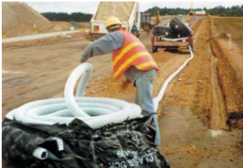
Figure 5.7: Drain pipe with pre-fitted sock being positioned
