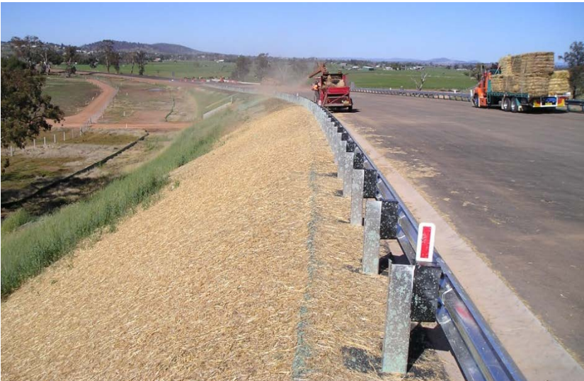
Figure 4.10: Progressive revegetation of an embankment with grass and straw mulch
