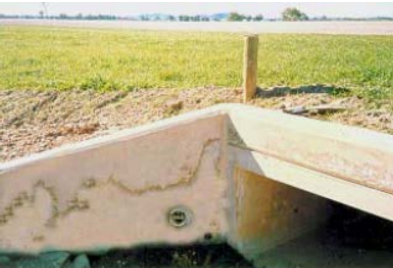
Figure 5.10: Subsurface drain outlet in culvert headwall
