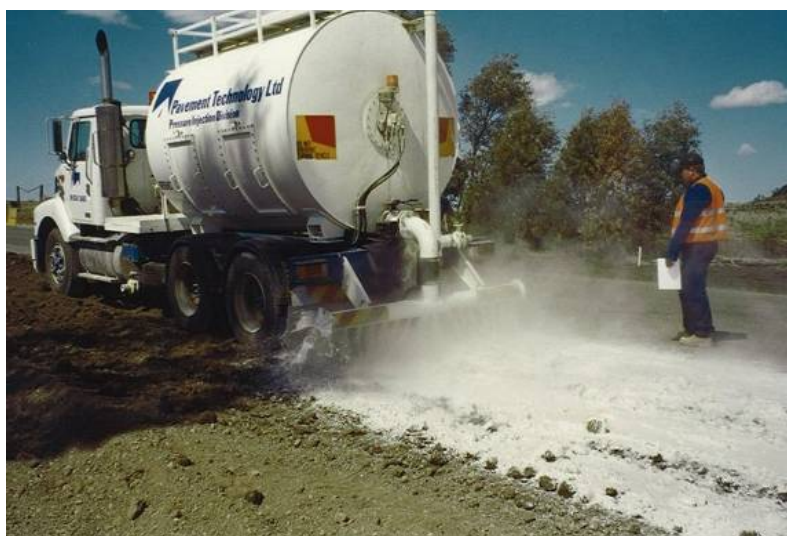
Figure 7.7: Lime slurry spreading
