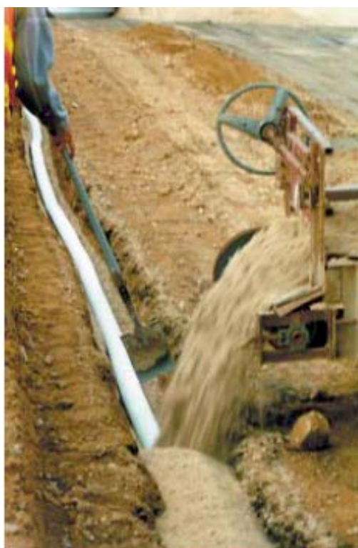
Figure 5.3: Placement of granular material
