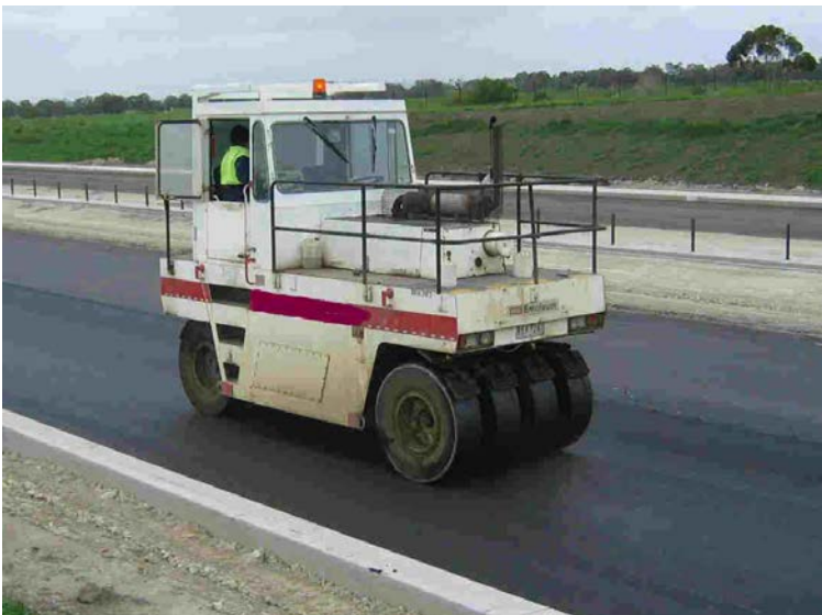
Figure 9.13: Pneumatic multi-tyred roller
