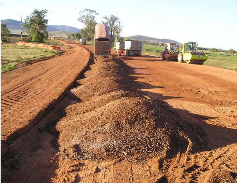
Figure 4.9: Dumping of material in heaps to be spread
