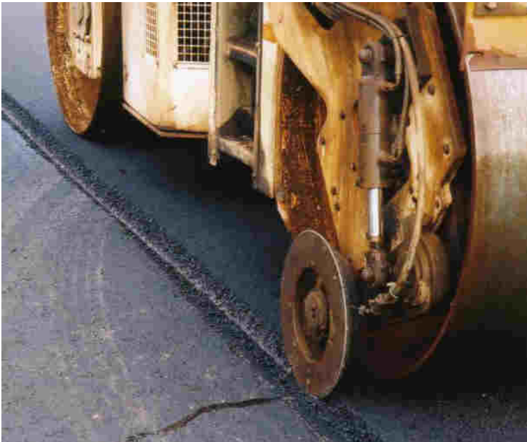
Figure 9.10: Cutting disc attached to steel roller
