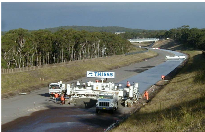
Figure 10.3: Tipper trucks being used on a typical PCP project
