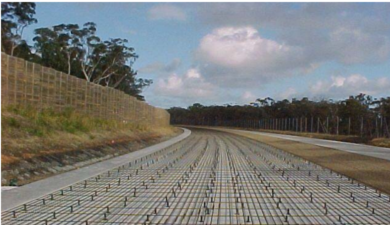
Figure 10.5: CRCP reinforcement
