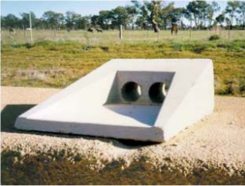
Figure 5.9: Pre-cast subsurface drain outlet
