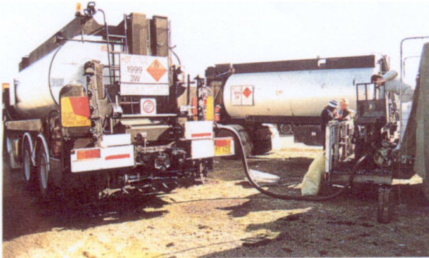
Figure 8.4: Road ranker (at rear) delivering binder to site
