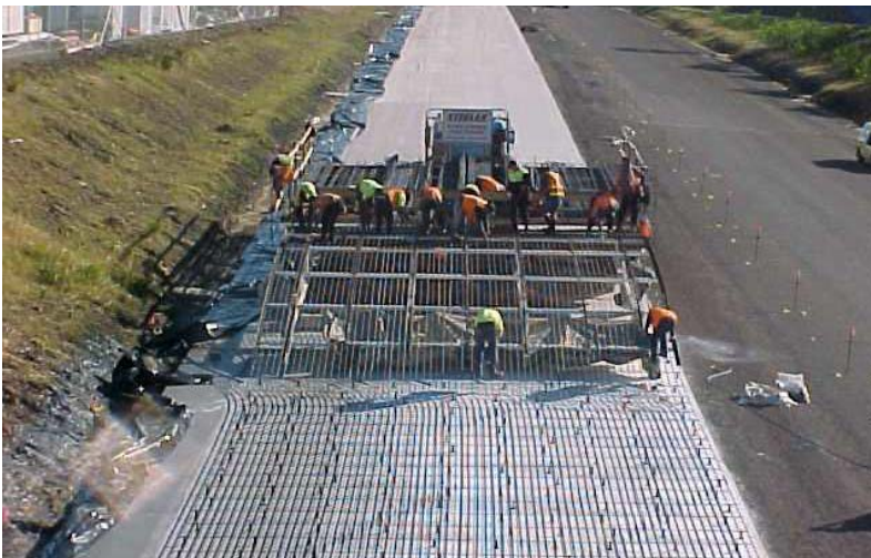
Figure 10.6: Erection of CRCP reinforcement
