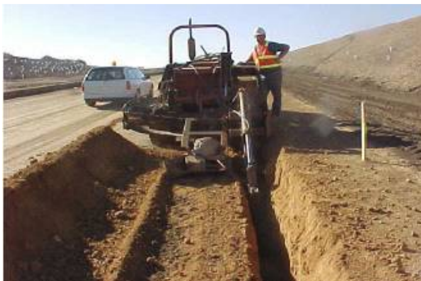
Figure 5.1: Trenching for subsurface drainage
