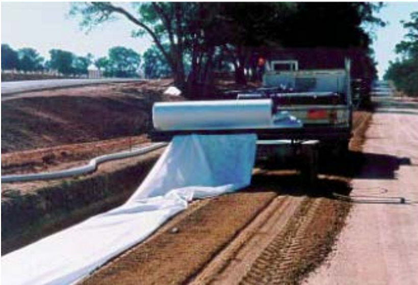
Figure 5.5: Placing a first-stage geotextile filter
