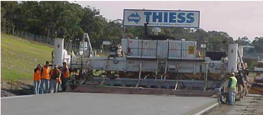
Figure 10.8: Slipform paver
