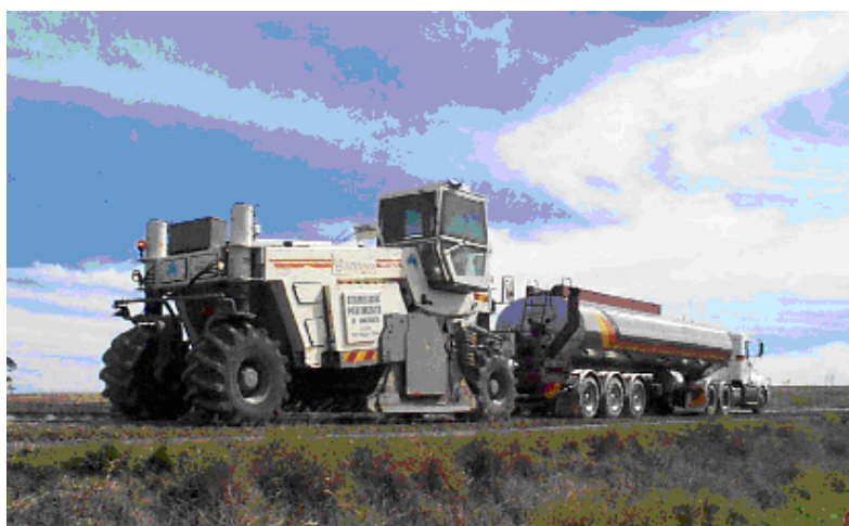
Figure 7.8: Liquid binder (foamed bitumen) added directly through recycler
