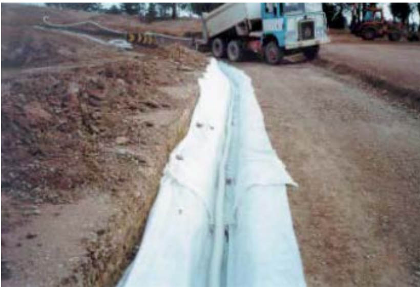
Figure 5.6: Discharge pipe in trench, ready for second-stage filter
