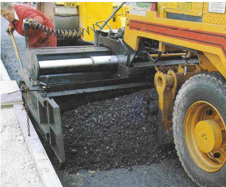
Figure 9.7: Paver with hydraulic screed
