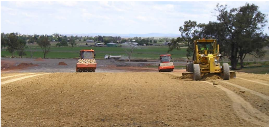
Figure 4.16: Compaction of an earthworks layer
