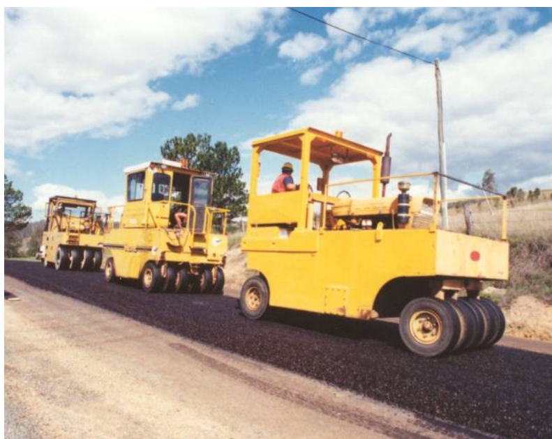
Figure 8.8: Pneumatic multi-tyred roller
