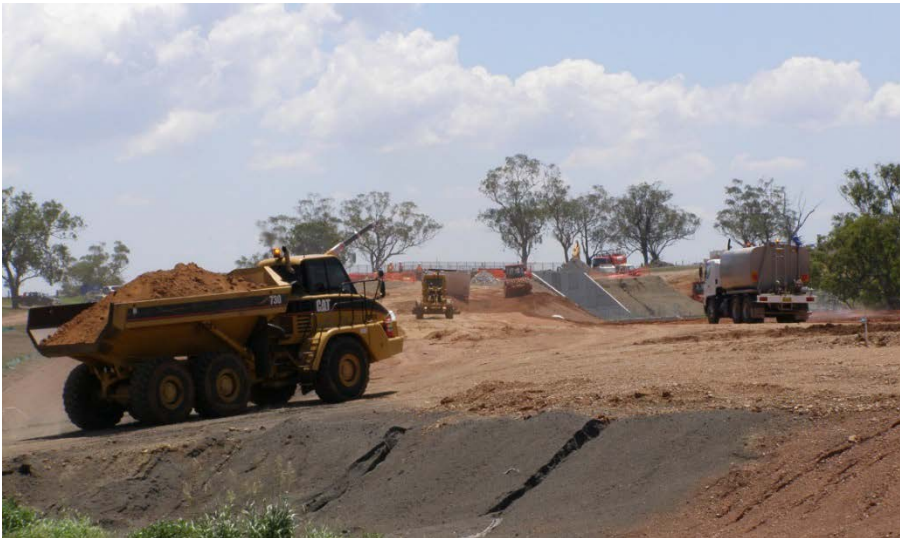
Figure 4.2: Dump truck delivering fill material
