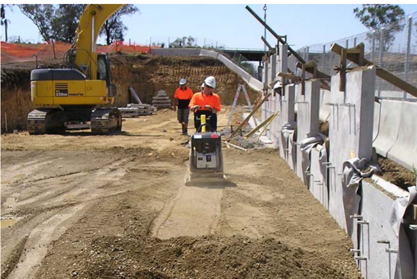
Figure 4.11: Hand compaction adjacent to reinforced soil wall
