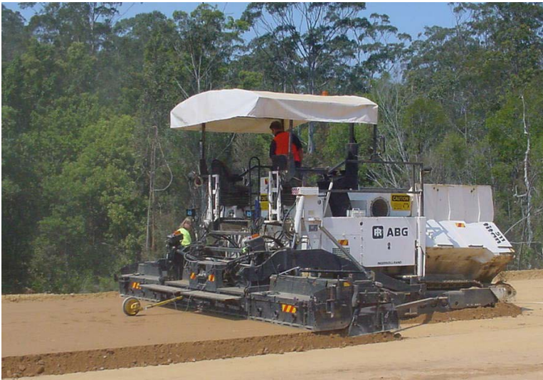
Figure 6.3: Paver laying granular material
