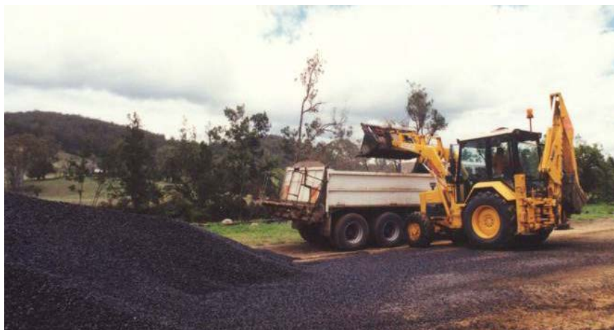
Figure 8.3: Loading precoated aggregate with a front-end loader
