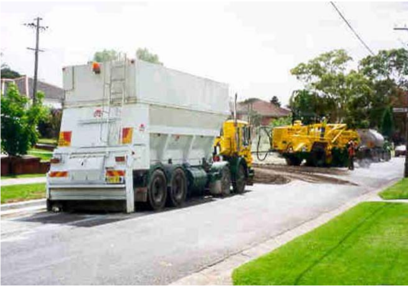
Figure 7.1: A mechanised spreader with rear drop chute
