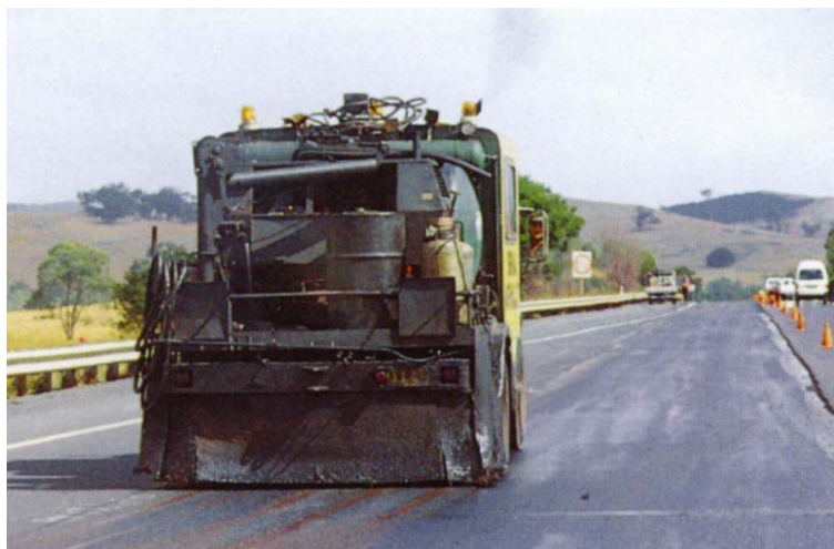
Figure 9.3: Tack coat sprayer in operation
