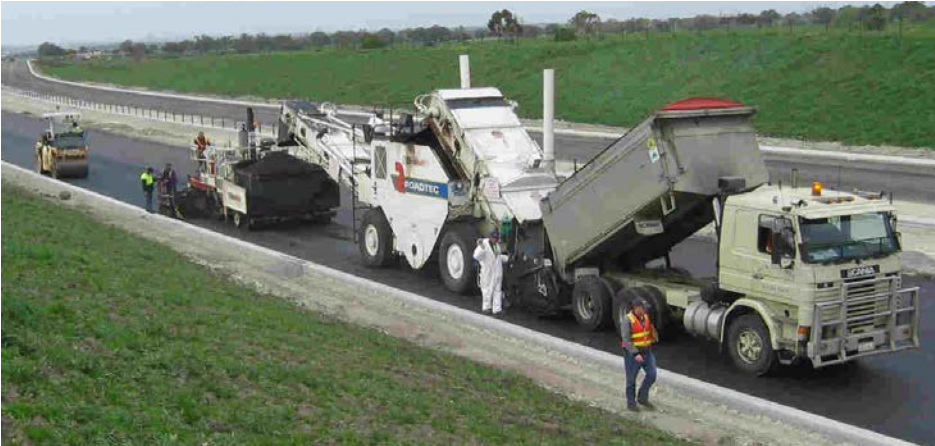
Figure 9.4: Materials transfer device
