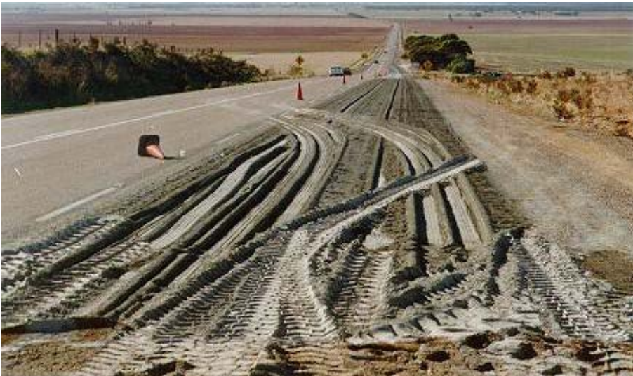
Figure 7.5 Construction traffic over spread binder may alter distribution
