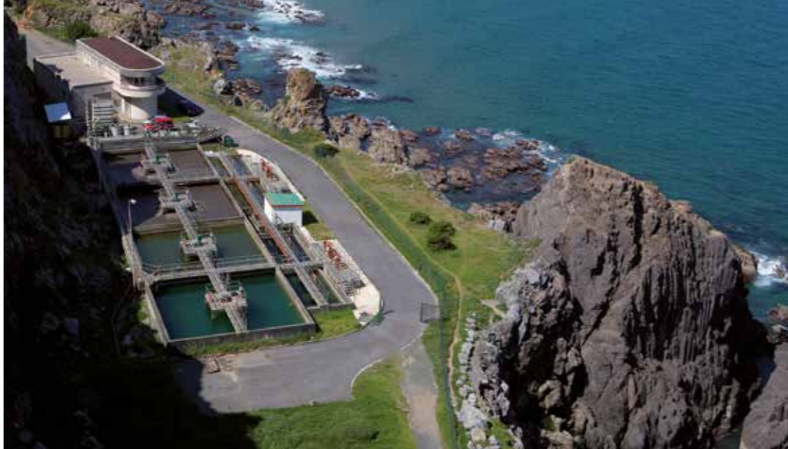
Bakio WWTP, Biscay, Spain
