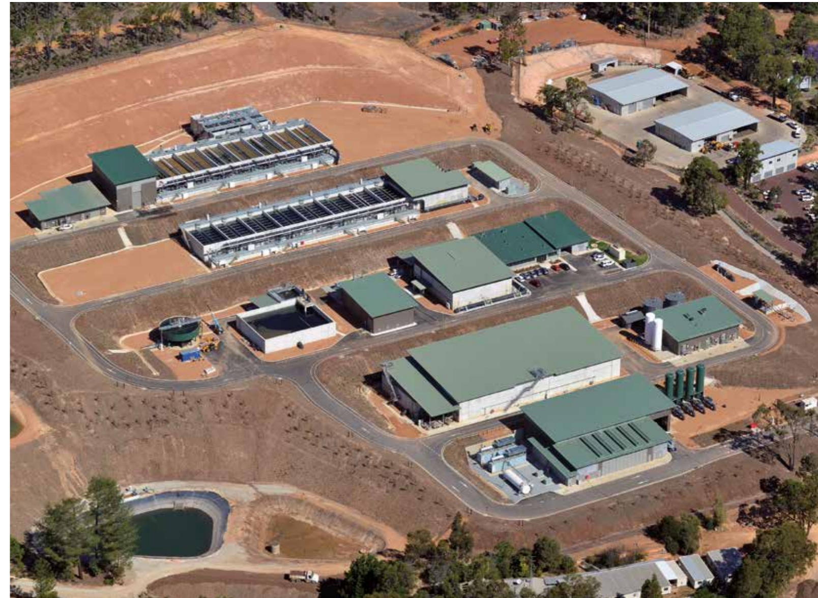
Mundaring DWTP, Perth, Australia
