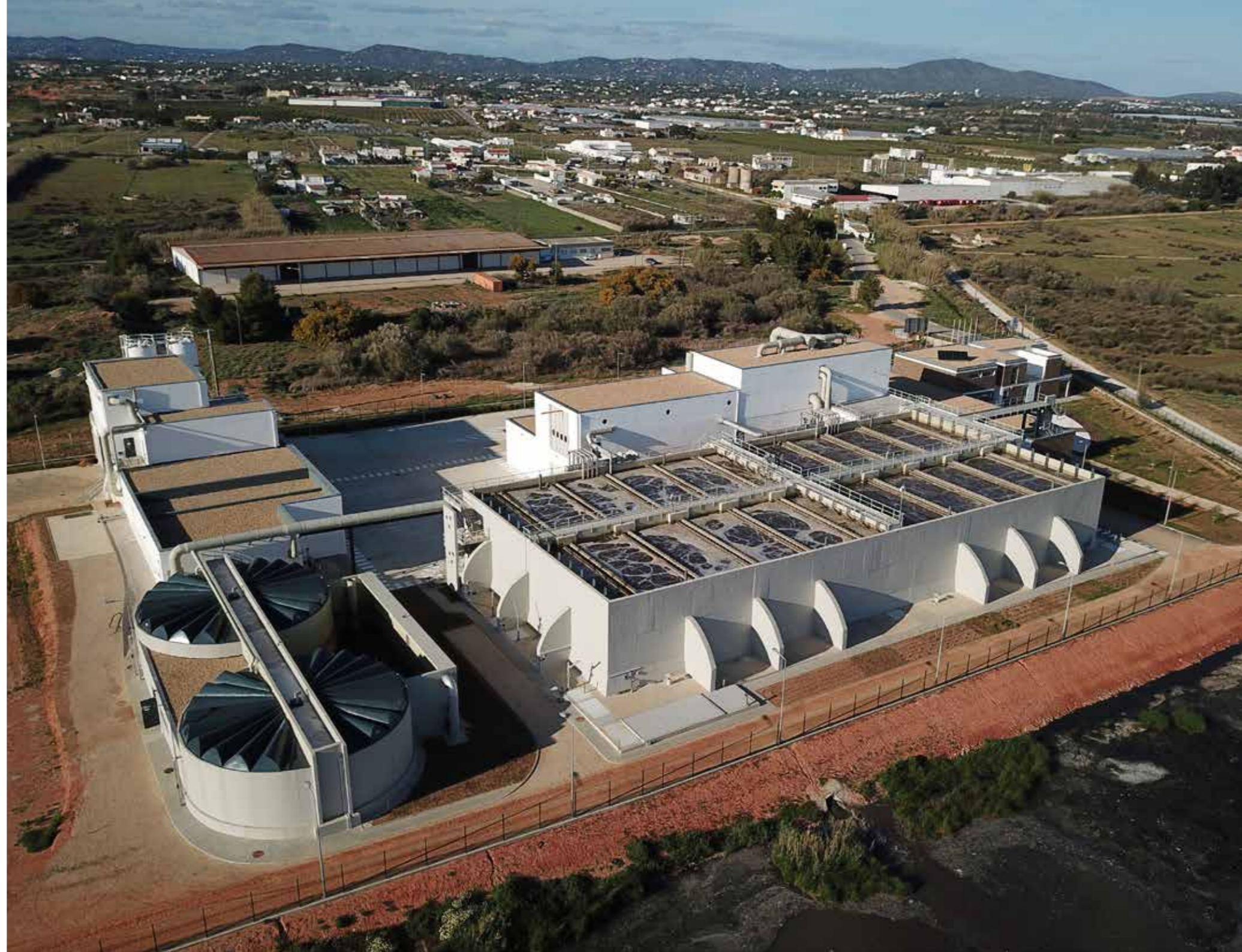
Faro WWTP, Algarve, Portugal
