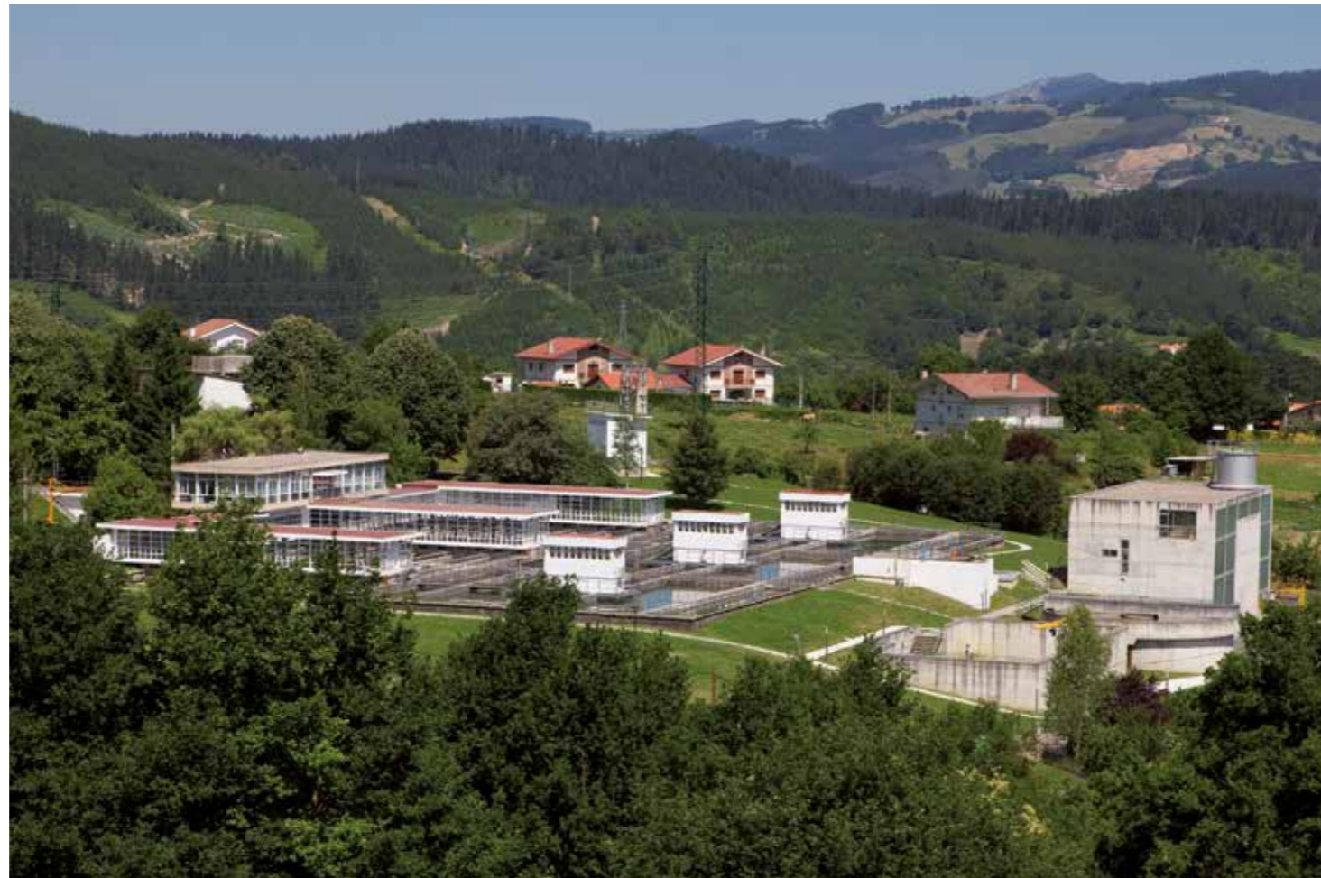
Sollano DWTP, Biscay, Spain
