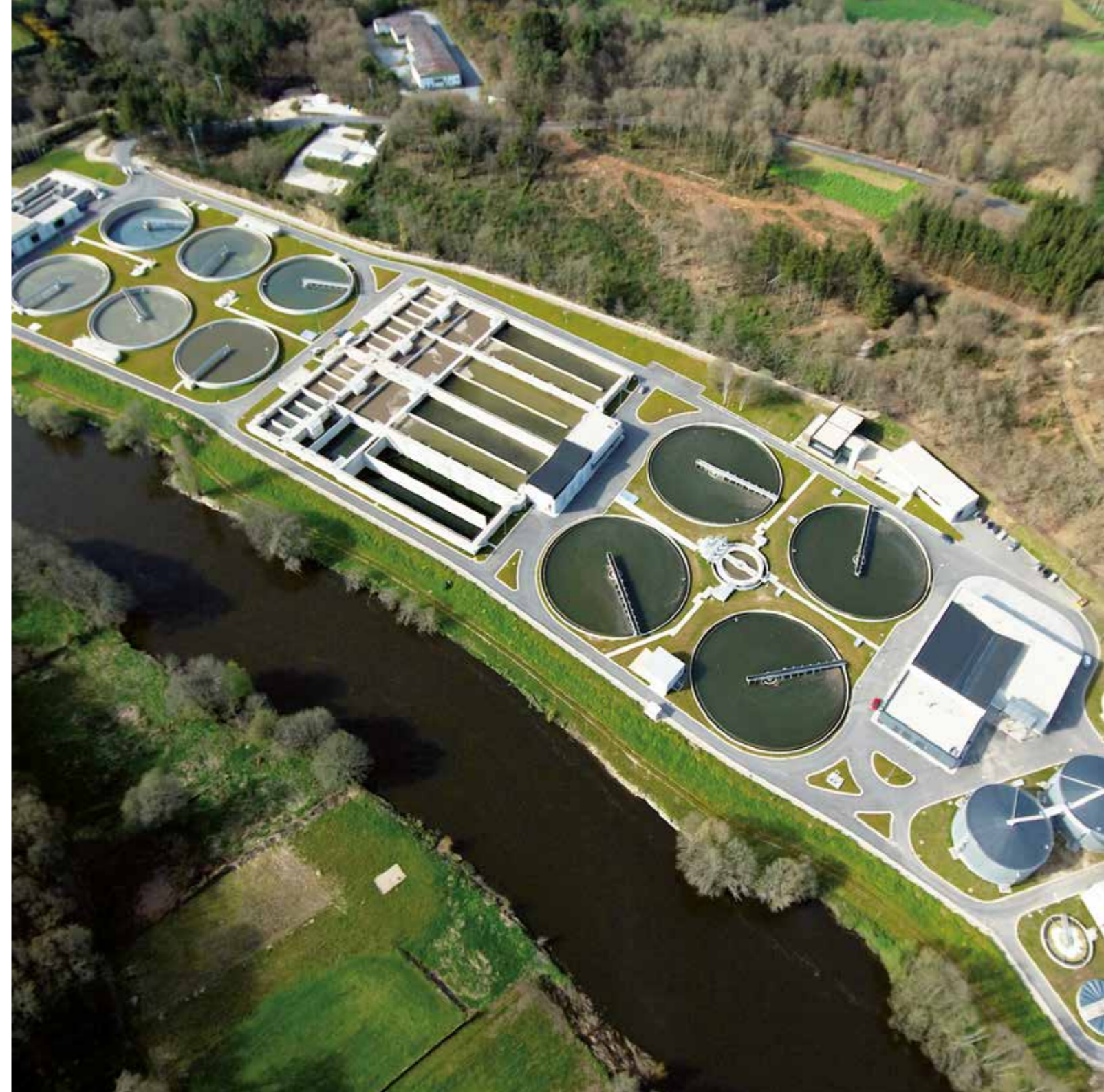
Wastewater treatment plant in Lugo, Spain
