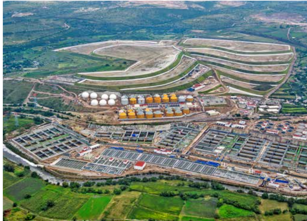
Atotonilco WWTP, Mexico
