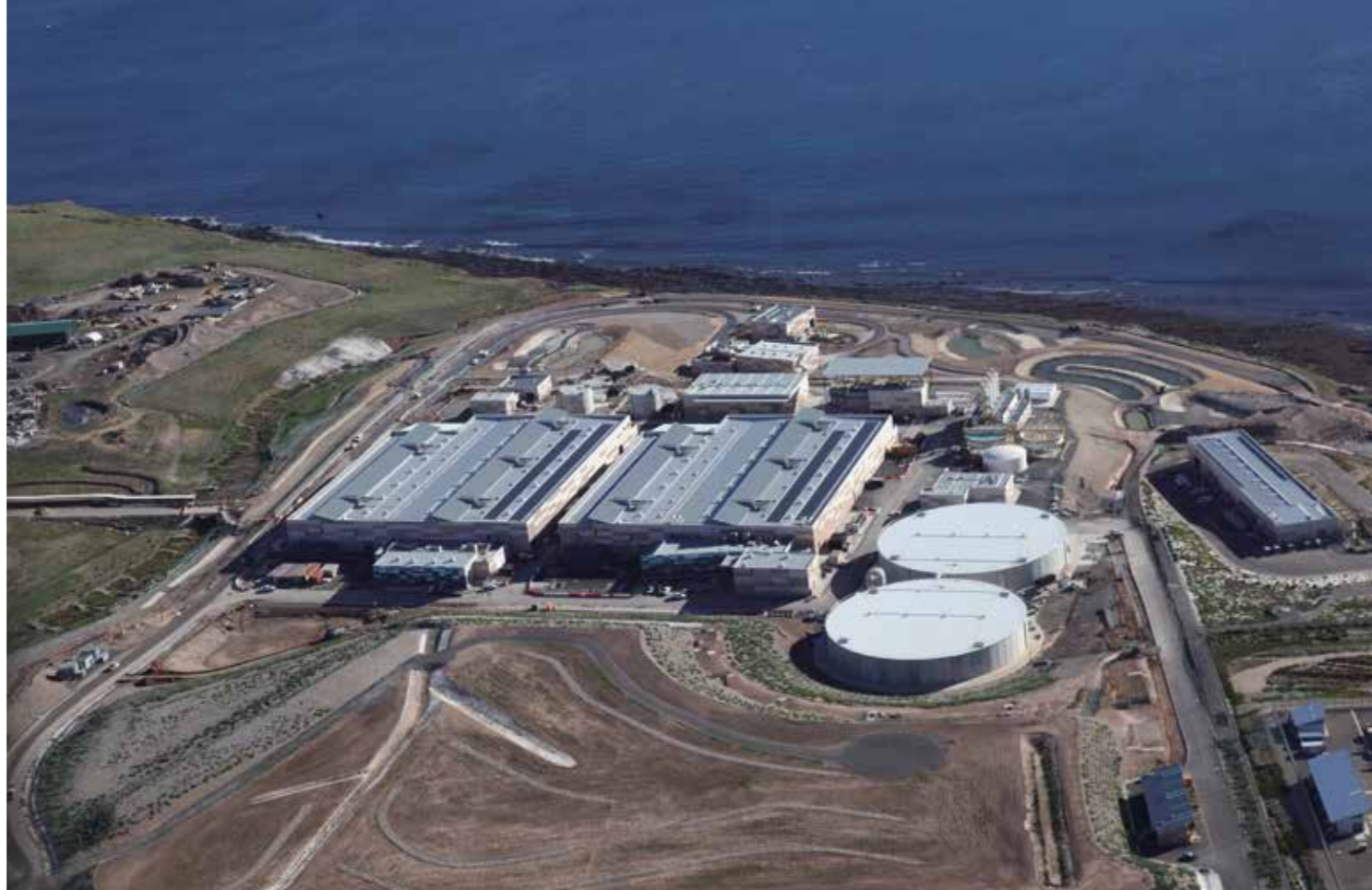
Port Stanvac desalination plant, Adelaide, Australia
