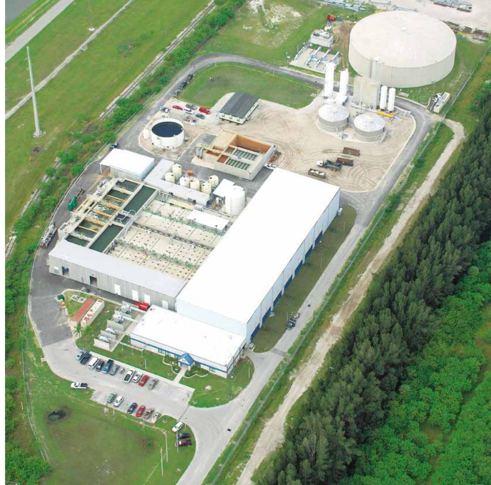
Tampa desalination plant, USA
