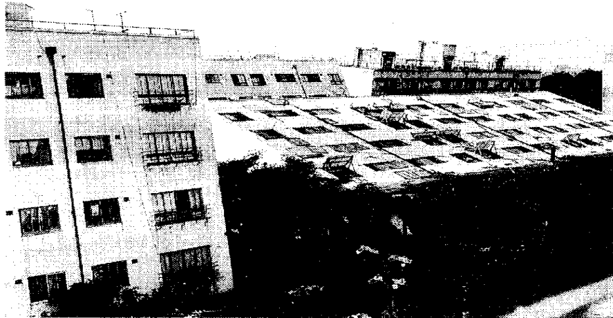
Phot. 8.1 Prefectural 4-story apartment houses of RC box-shaped wall building in Kawagishi-cho, Niigata City, which turned over in the Niigata Earthquake in June 1964
