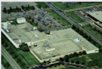
Global headquarters of McQuay (Minneapolis, USA)
