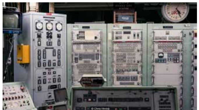
Titan II Control Center
