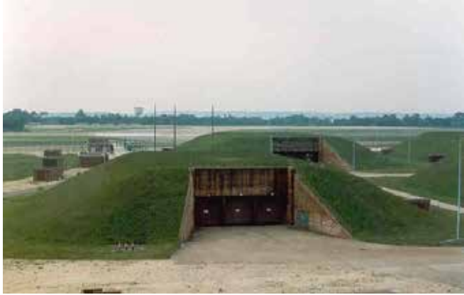
GLCM Alert and Maintenance Area
