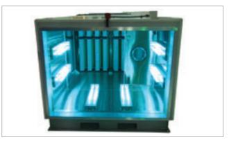
Ultraviolet air sterilization within the air handling unit
