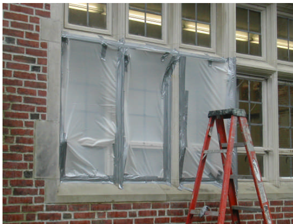
Photo 3 – Window from Photo 1 sealed on exterior for chamber air leakage measurement
