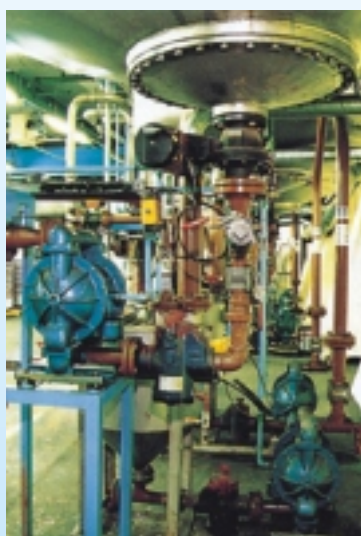
Part of the filtration process at a major multi-national paint manufacturer where Blagdon 50 pumps are used to supply the fully automated filling line.
