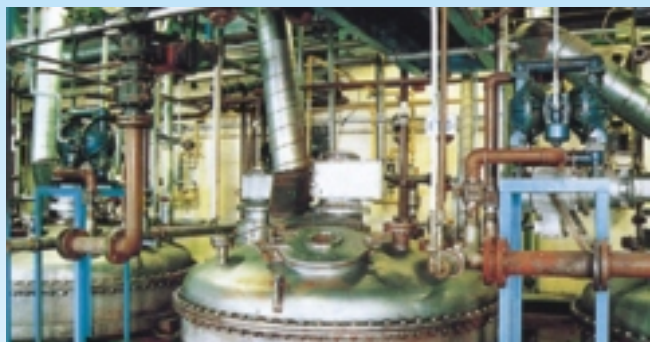
Blagdon 50 pumps feeding a ring main for final blending at a coatings producer.
