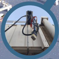
Cables for aircraft ground power
