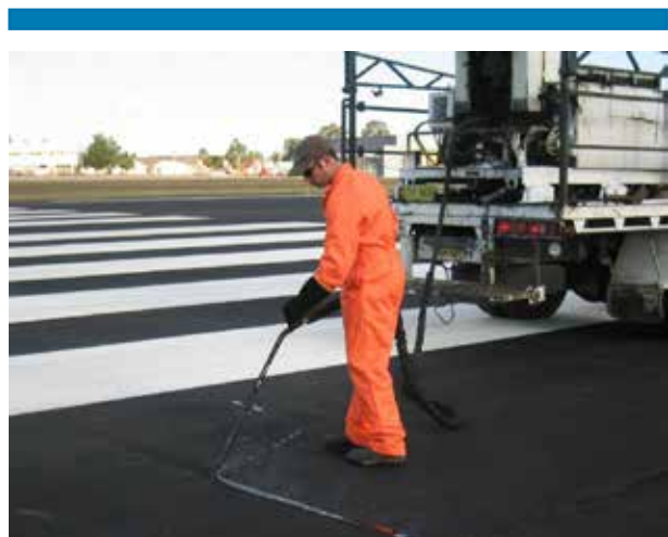
Figure 44: Hot bitumen crack bandage application
