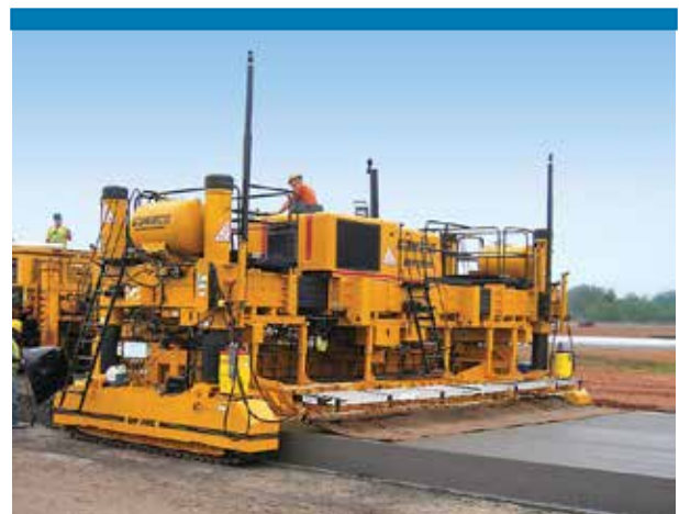
Figure 36: Slip form paving rigid airfield pavement (Hodgkinson 2016)
