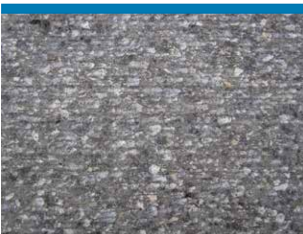
Figure 33: Milled and cleaned asphalt surface
