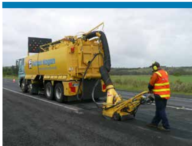
Figure 44: Hot bitumen crack bandage application
