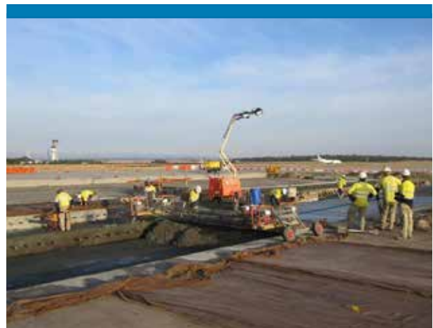
Figure 36: Slip form paving rigid airfield pavement (Hodgkinson 2016)
