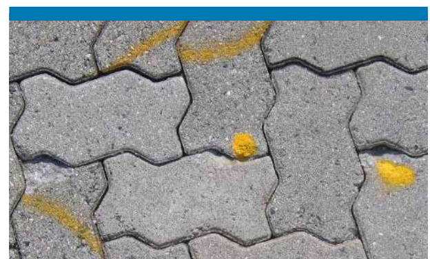
Figure 18: Concrete block pavers on a flexible airport pavement
