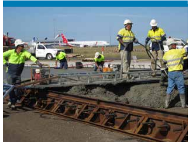
Figure 35: Infill paving of concrete with single-sided form
