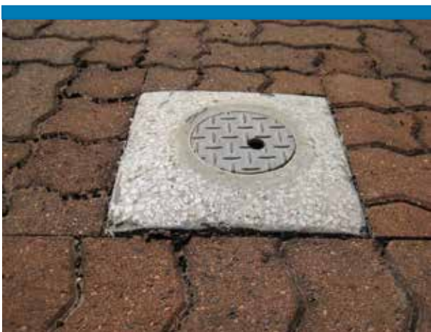
Figure 39: Multiple large part-blocks to avoid small part-blocks and slithers
