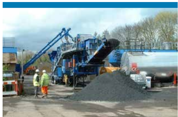
Figure 31: FCR moisture addition in an on-site pug mill
