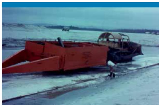
Figure 28: Flooded sand compaction
