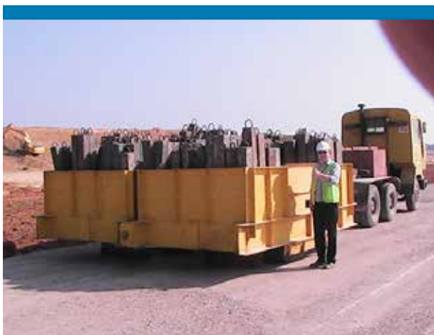
Figure 41: 50 tonne Marco roller
