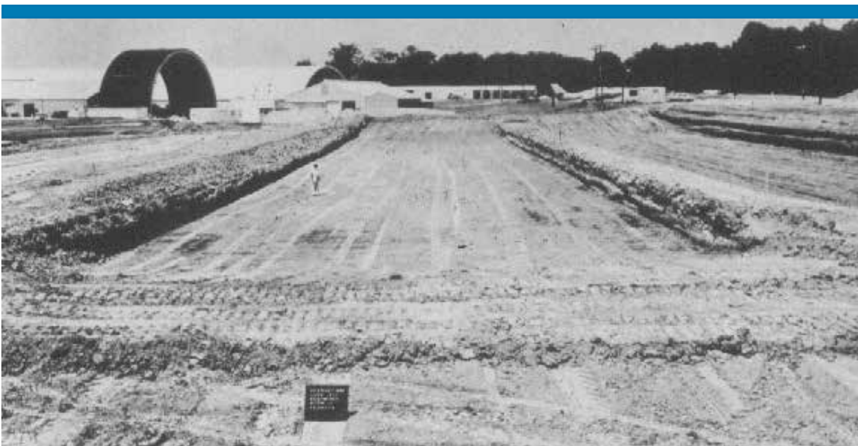
Figure 22: Example of US Army Corps pavement test section
