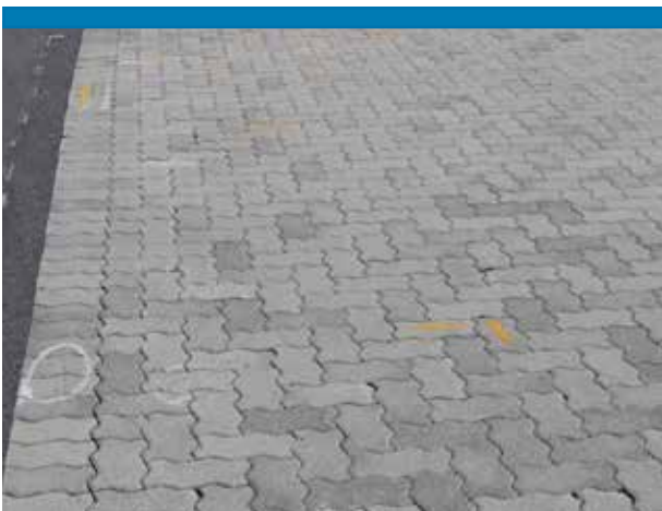
Figure 39: Multiple large part-blocks to avoid small part-blocks and slithers
