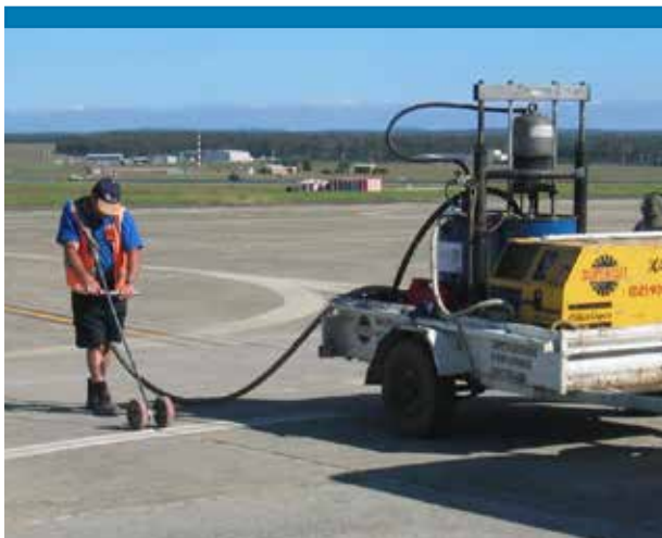
Figure 47: Joint sealant replacement
