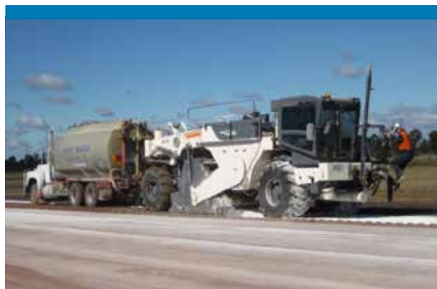
Figure 29: Insitu lime stabilisation
