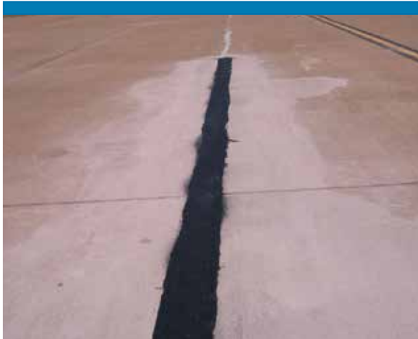
Figure 46: Semi-rigid epoxy spall repair
