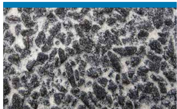
Figure 16: Example sprayed seal surface suited to a runway
