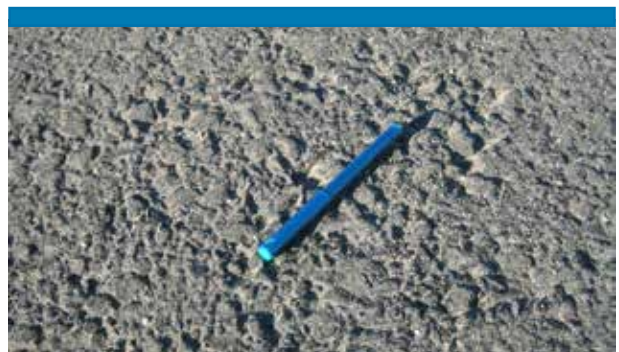
Figure 48: Isolated segregated asphalt treated by surface filling product
