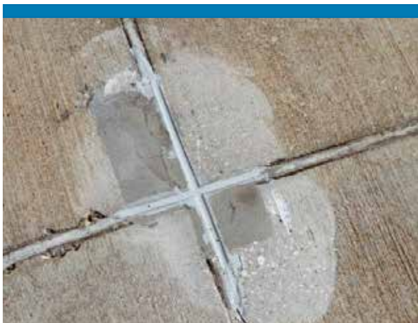
Figure 47: Joint sealant replacement
