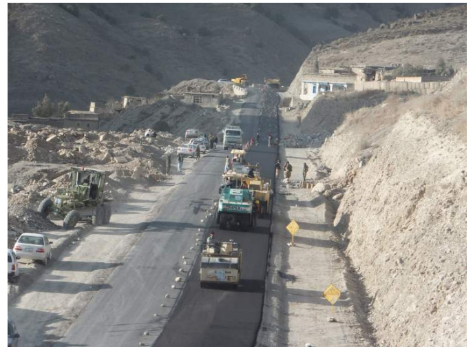
Gardez-Khost Highway under construction (USAID)
