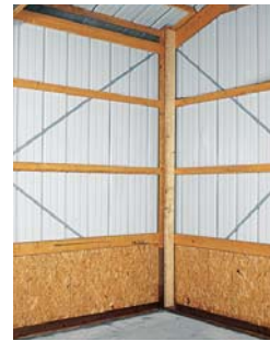
View of corner section before insulation
