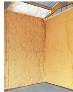
Add blankets of insulation and air deflector
