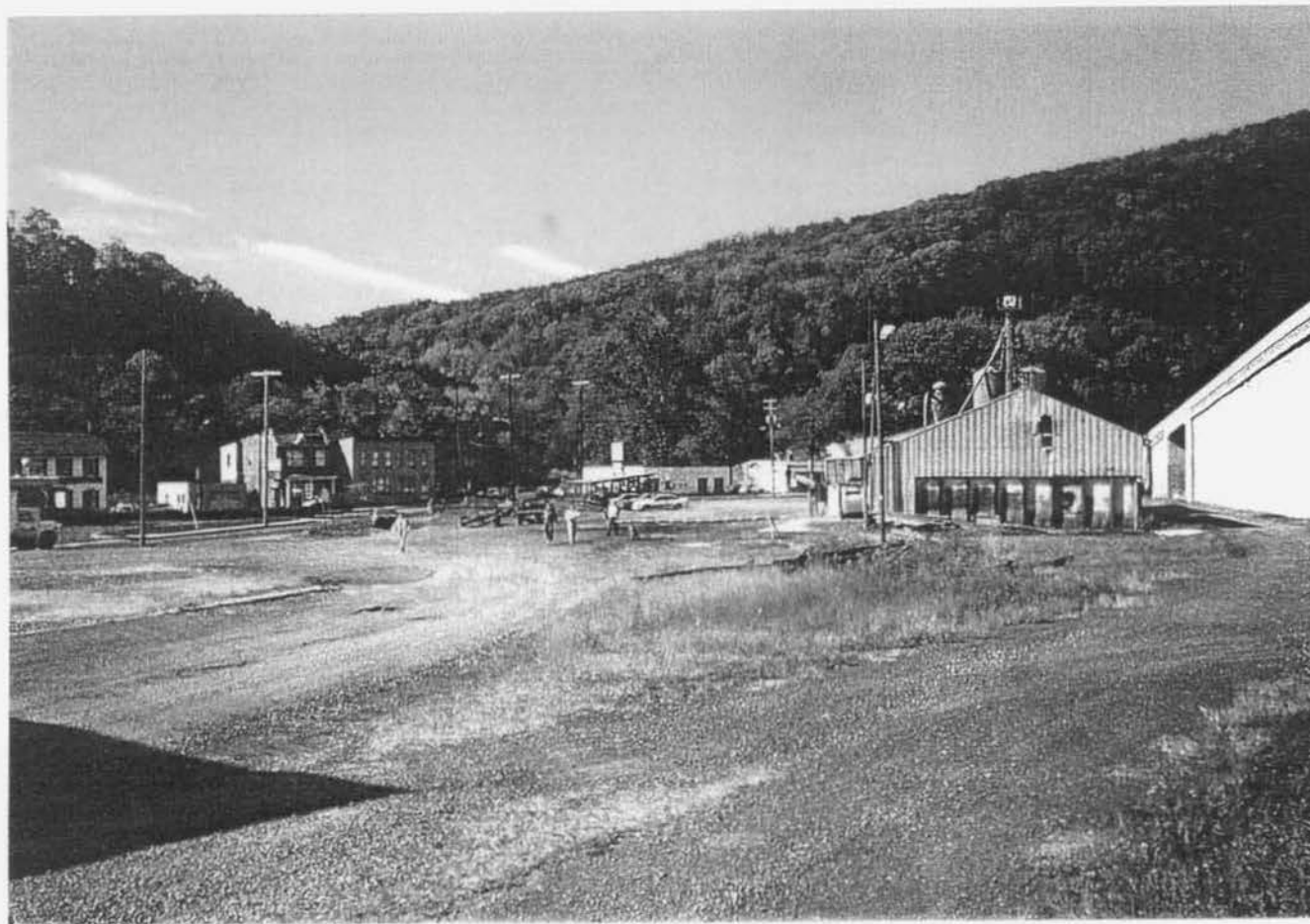
Former Track Roadbed/Alignment @ Southern States (looking west)
