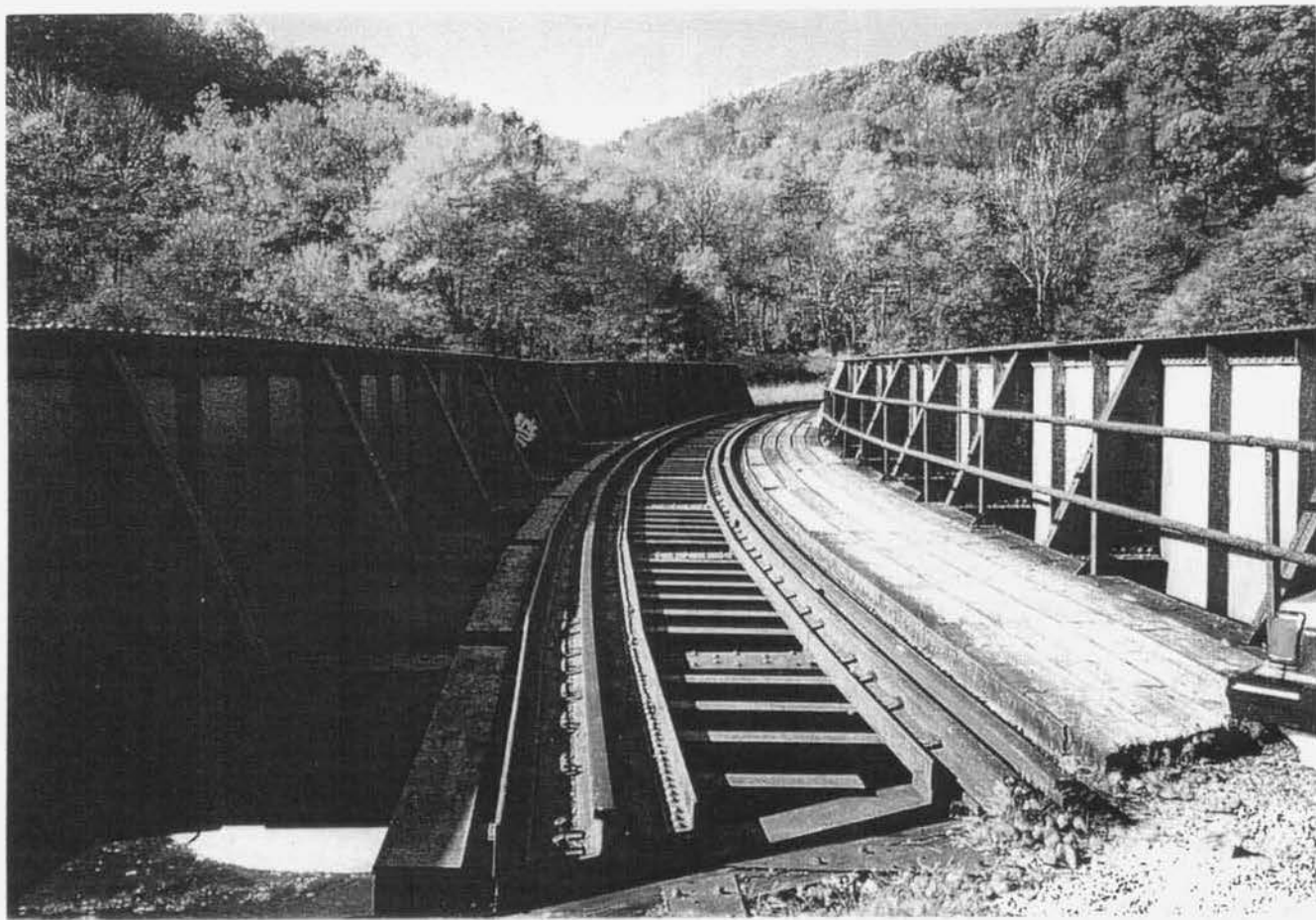
Tracks on Bridge (looking west)
