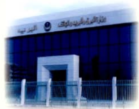
Post Office Building in Al Khobar
