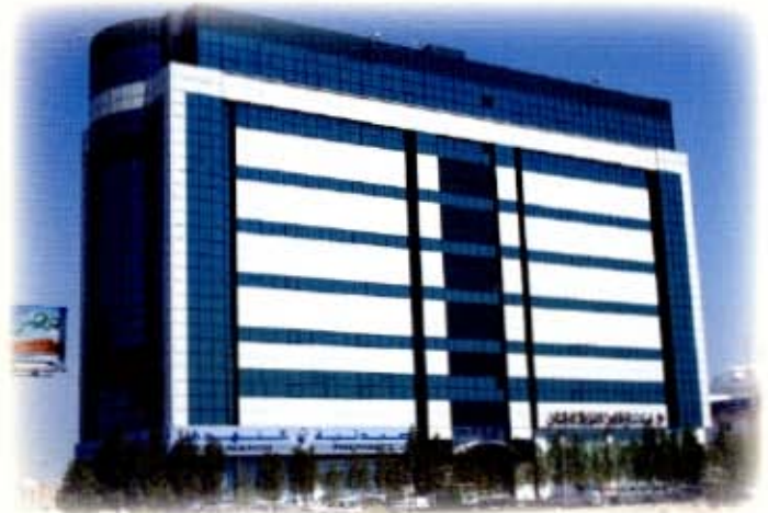
Al bahrain building in Al Khobar
