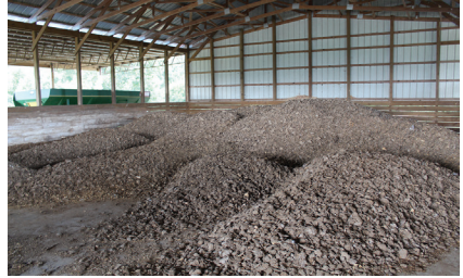
Figure 2. Manure storage in covered system.
