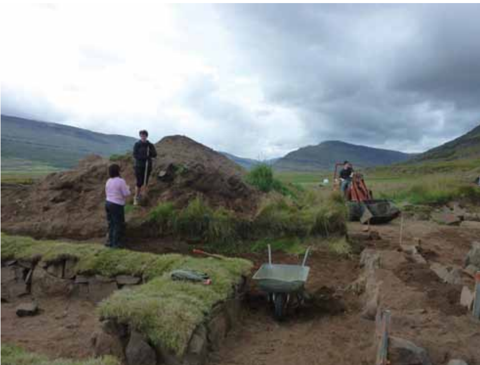
Small mountains of earth also were shoveled by hand and wheeled into the excavation area to restore the monastery rooms. Lower left, the beginnings of interior Icelandic rock-and-earth walls constructed by the volunteers. In background, view of the Fljótisdalur Valley of East Iceland.
