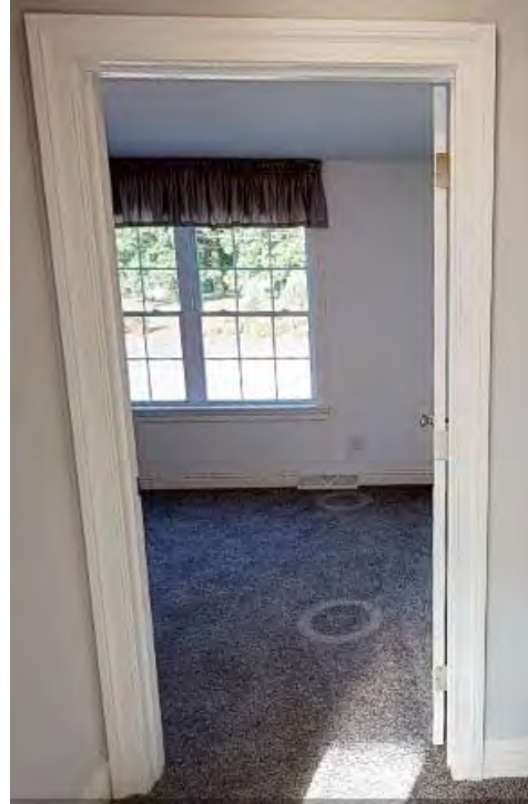
3 ¼" Casing, 5 ¼" Base White MDF Molding Or Opt. White Painted Pine ($$$)
