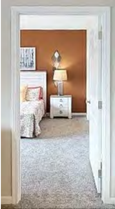
2 ¼" Casing, 3 ¼" Base White Colonial MDF Molding (Std Lifestyle) Or White Painted Pine (Std Classic Series)
