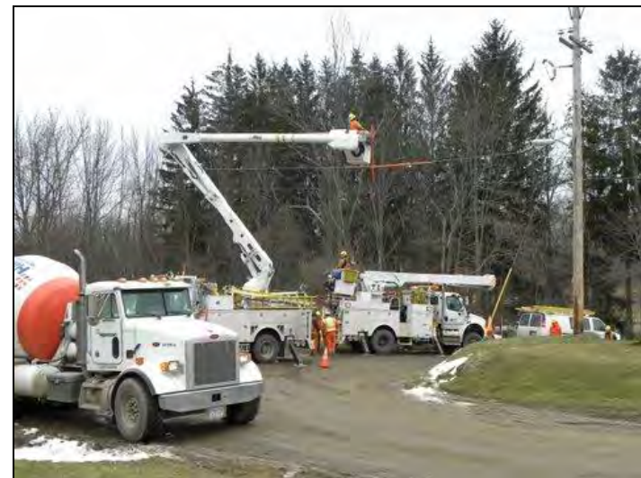
Electric Line Workers
