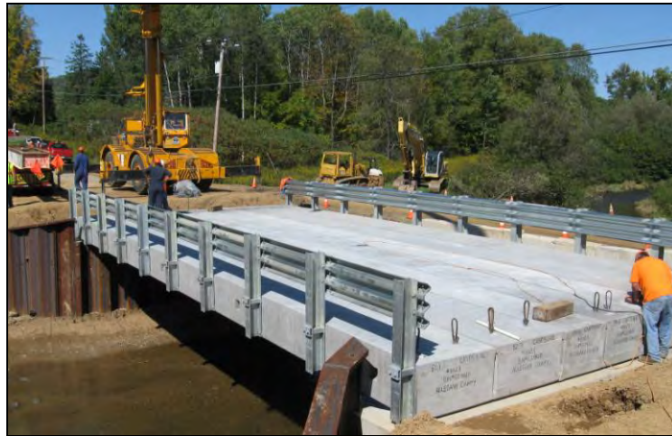
New Bridge Installation
