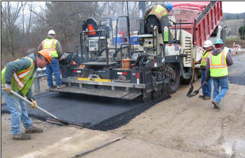
County Crew Bridge & Paving Project
