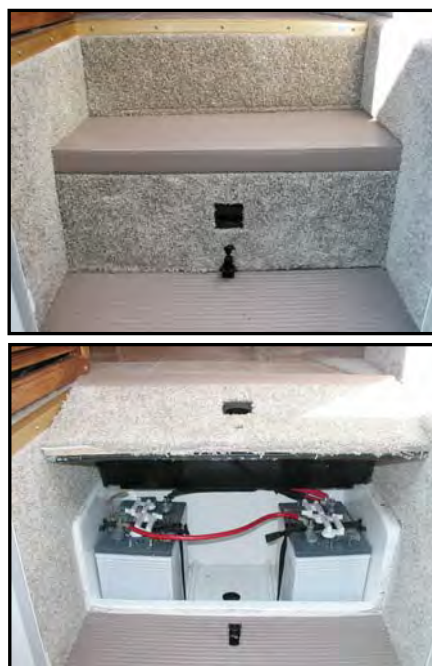
Figure 7-3. Stairwell (Top) and Battery Storage Underneath (Bottom)
