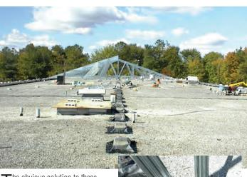
The obvious solution to these retrofit challenges was a sloped roof with a built-in mechanical space. Although the traditional approach would have been to utilize a structural "post and purlin" system, the architect wanted to ensure suffi-
