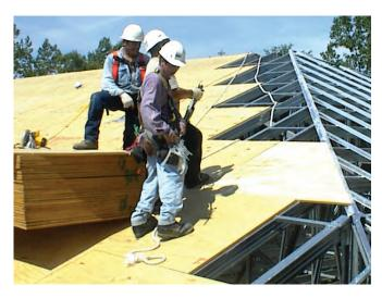
The STABILIZER® not only spaces trusses and braces, but can remain in place as roof sheathing is applied. This is just one more way to save money on your project.
