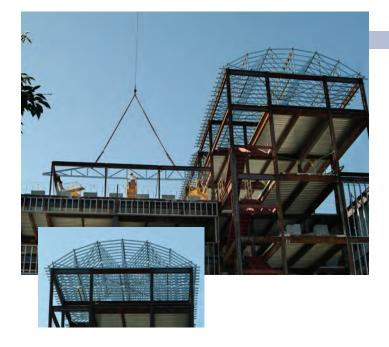
This truss profile employs both a radius top, and built-in gutter detail.
