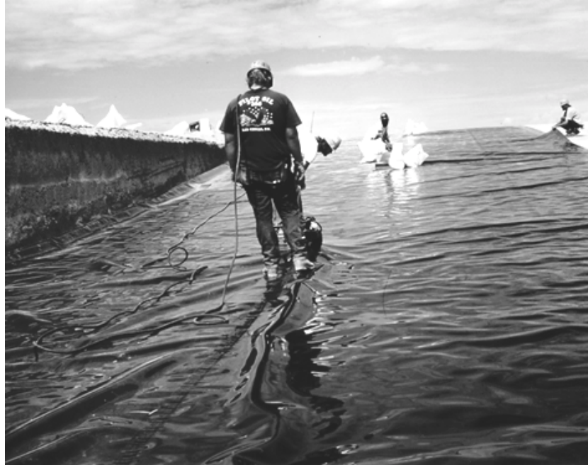
Figure 6. Welding seams of geomembrane panels, RCRA Subtitle C.
