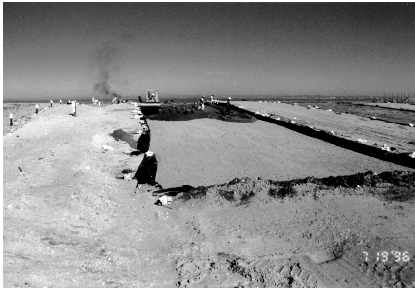
Figure 12. Anisotropic barrier installation.
