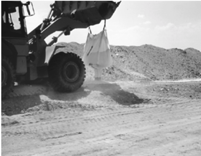
Figure 4. Adding sodium bentonite to native soil, RCRA Subtitle C.
