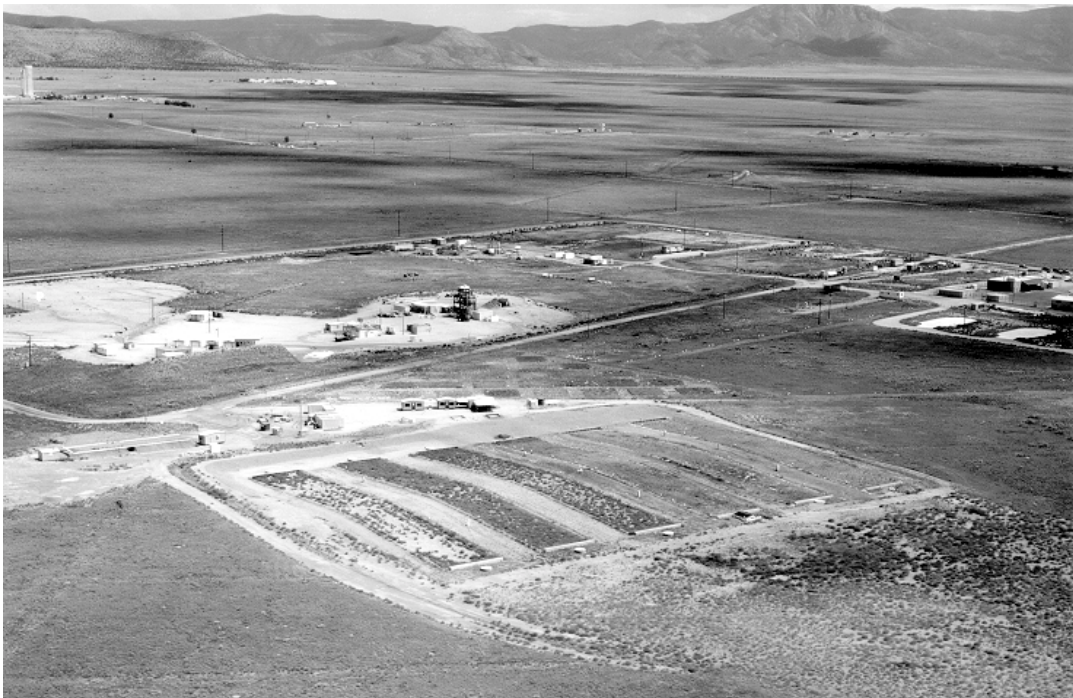
Figure 1. Aerial view of alternative landfill cover demonstration.
