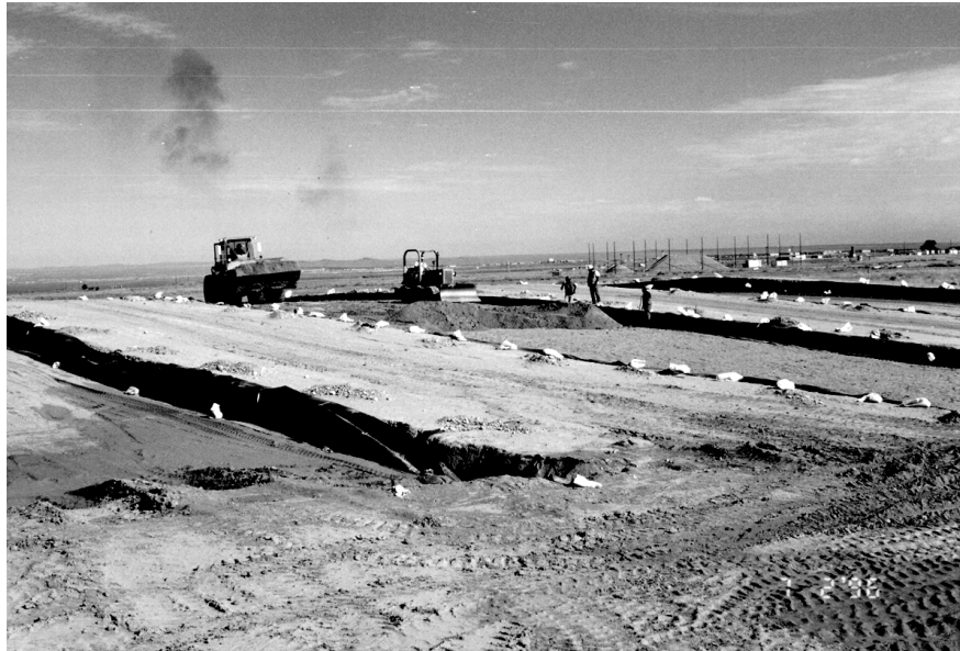
Figure 10. Capillary barrier installation.
