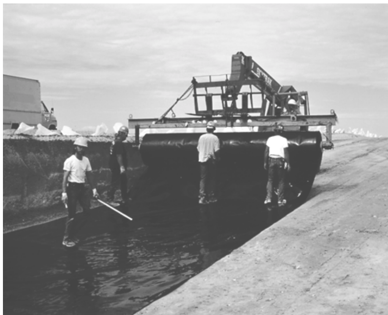
Figure 5. Geomembrane placement with spreader-bar attachment, RCRA Subtitle C.
