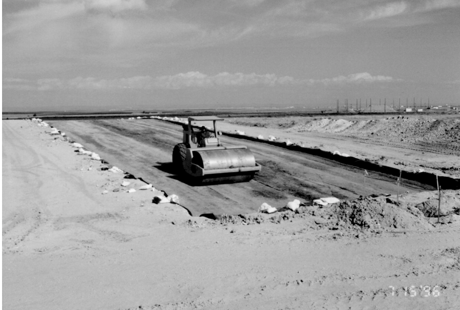
Figure 14. Compacting soil in ET cover.
