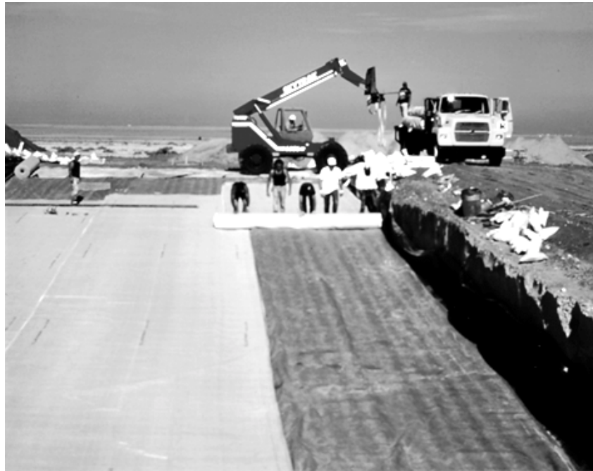
Figure 8. GCL installation.
