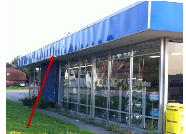
Flat-sheet aluminum displaying oil-canning
