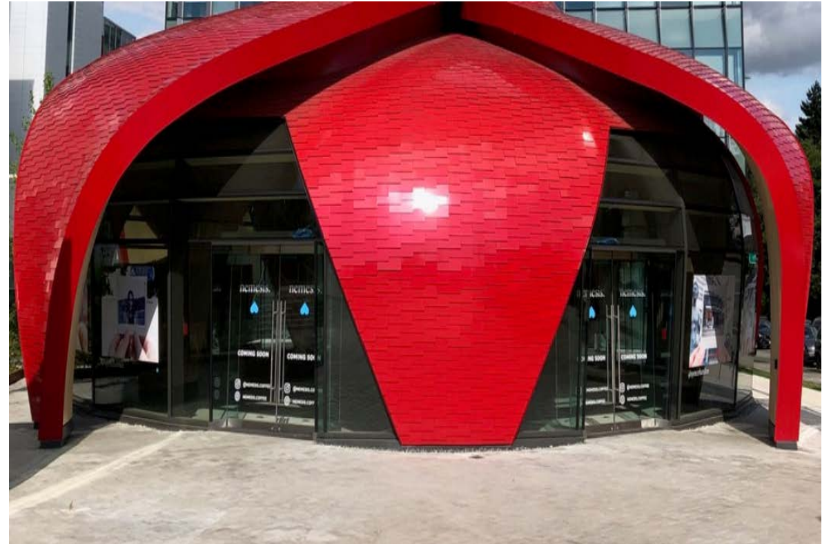
Designed by Perkins + Will, 569 Great Northern Way was part of a larger redevelopment project at the Emily Carr University of Art & Design in Vancouver, British Columbia. The 3,000-square-foot building is clad in a custom color-shifting paint finish.
