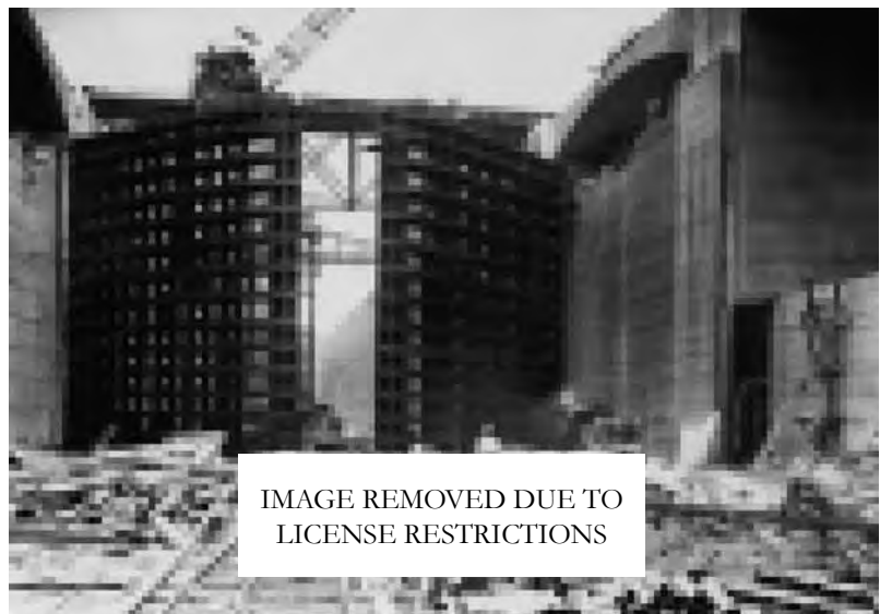
Construction of Locks for the Panama Canal, April 5, 1913
