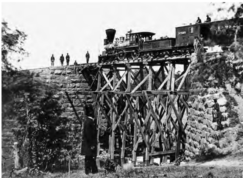
Orange and Alexandria Railroad Military Bridge
