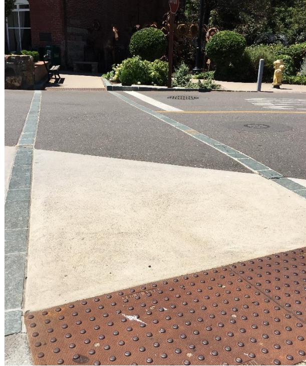
Figures 13&15. Amador City's rust colored ADA curb ramps and stone pedestrian crossing.
