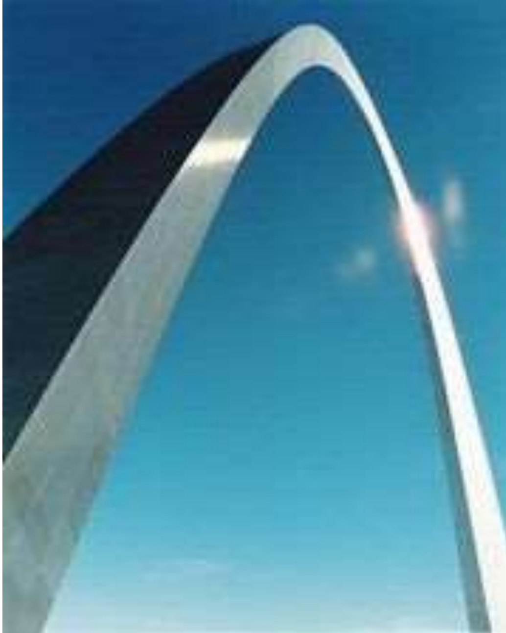
The 630-foot (192 m) high, stainless-clad (type 304) Gateway Arch defines St. Louis's skyline.
