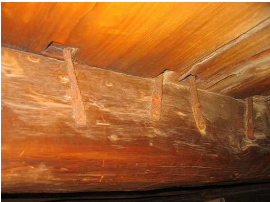
The Nightingale Floor construction.
