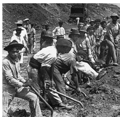
▲ Workers digging the Panama Canal faced hazardous landslides and death from disease.
