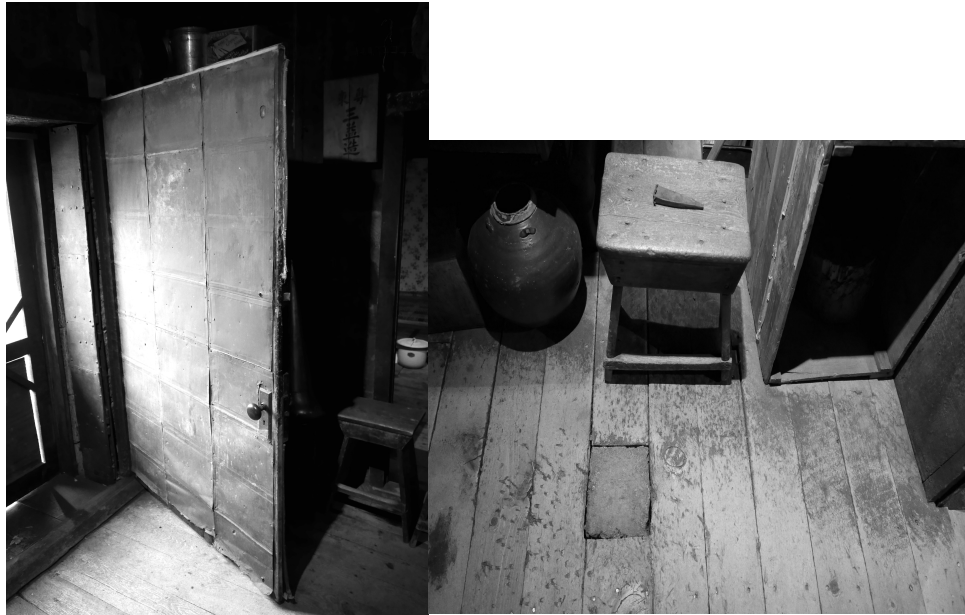
Fig. 2.1 Fortified Door and Wooded Block Embedded in the Floor at Kam Wah Chung
