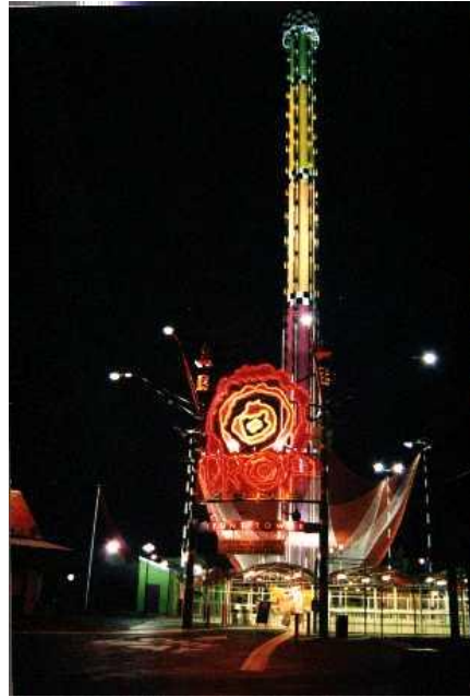
Drop Zone, Paramount Great America Electrical design for ride power & controls connections as well as tower and site lighting. The tower lighting was required to comply with FAA regulations.
