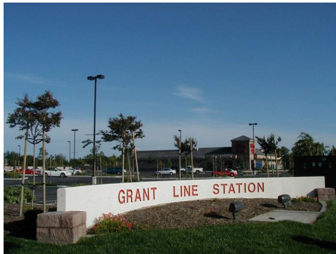
Commercial Center – Tracy, CA Provided electrical design for site lighting and utilities extension to new commercial spaces.
