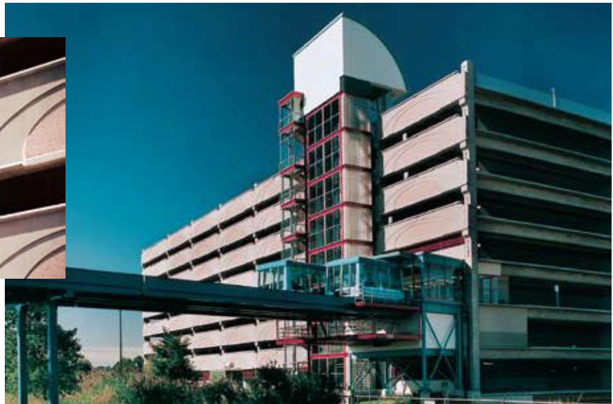
Mystic Transportation Center, Medford, Mass.; Architect: Thompson Design Associates.
