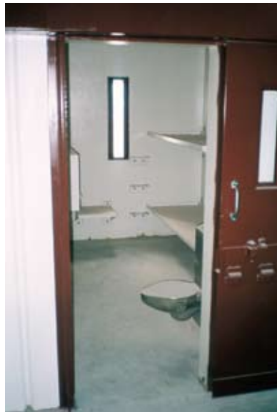
The cells arrived at the job site with furnishings, light and plumbing fixtures, windows, and door frame.
