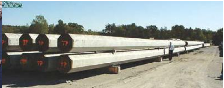
Bath Iron Works Land Level Transfer Facility, Bath, Maine; Design-Build: Clark Group.
