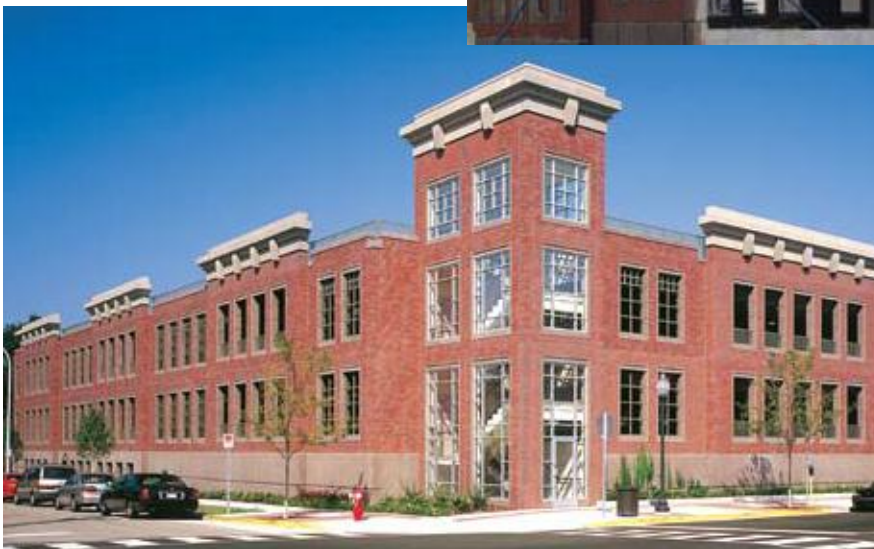
Fifth & Lafayette Parking Structure, Royal Oak, Mich. The exterior façade combines 173 different shapes of brick clad lite walls. The lite walls are used to replicate the appearance of windows.
