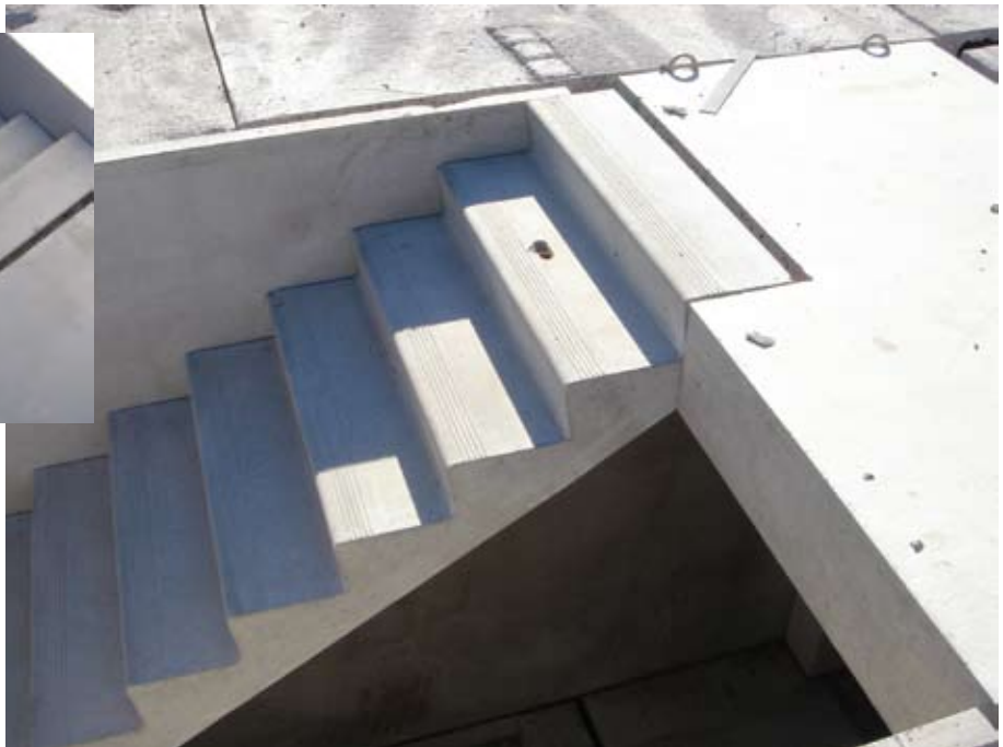
Stair run supported by precast concrete landing.
