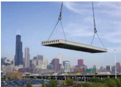
Hollow-core plank. Photo: The Spancrete Group.
