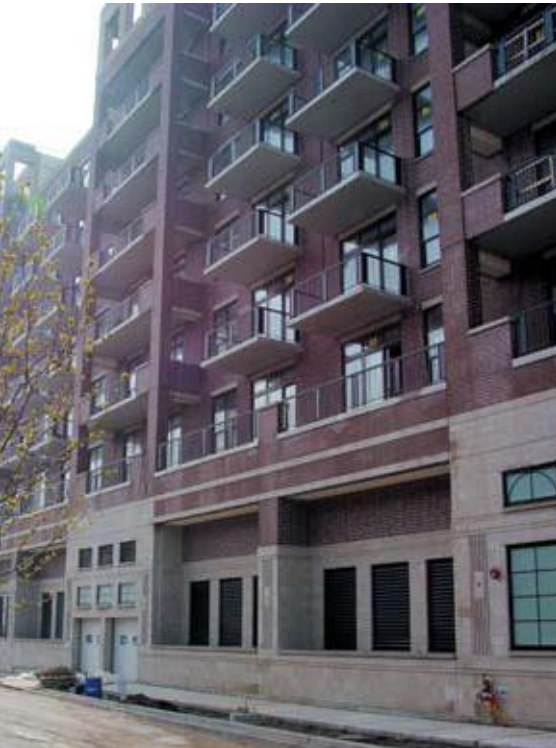
Precast balconies alternate with porches along the building façade to create a dynamic rhythm.
