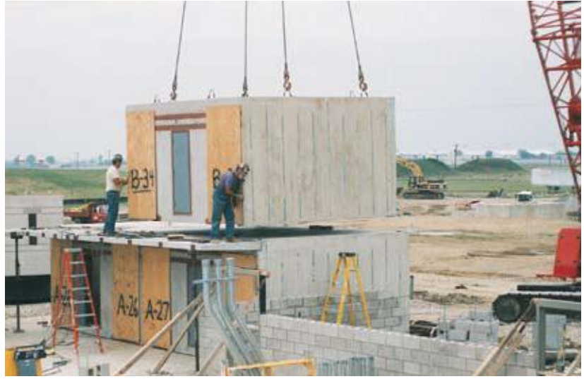
A crane lifts a 44,000 lb modular cell unit into place, forming the second level of one of the Medium Housing Buildings.
