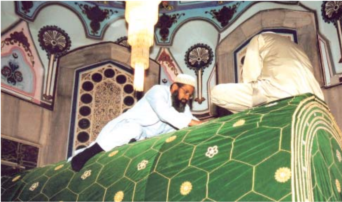
Above: Completing the installation of the covering.
