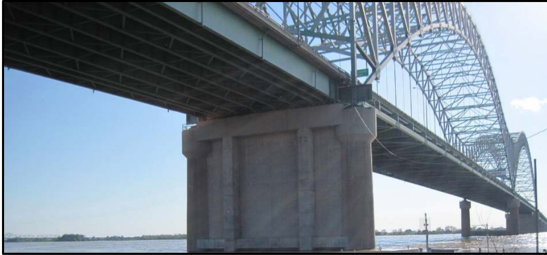
Figure 7.13 - Substructure at Pier C
