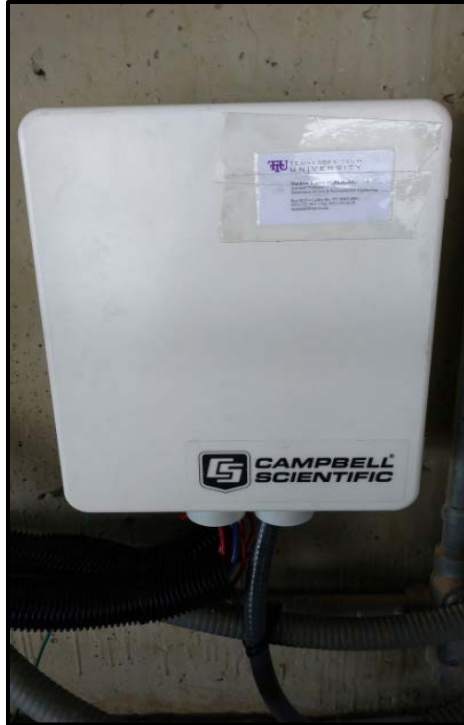
Figure 6.5 - Box C Post Installation
