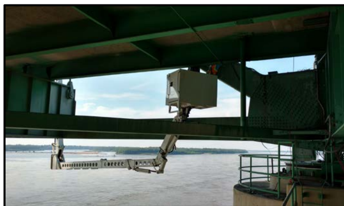
Figure 6.2 - Snooper Truck Use during Strain Gage Attachment
