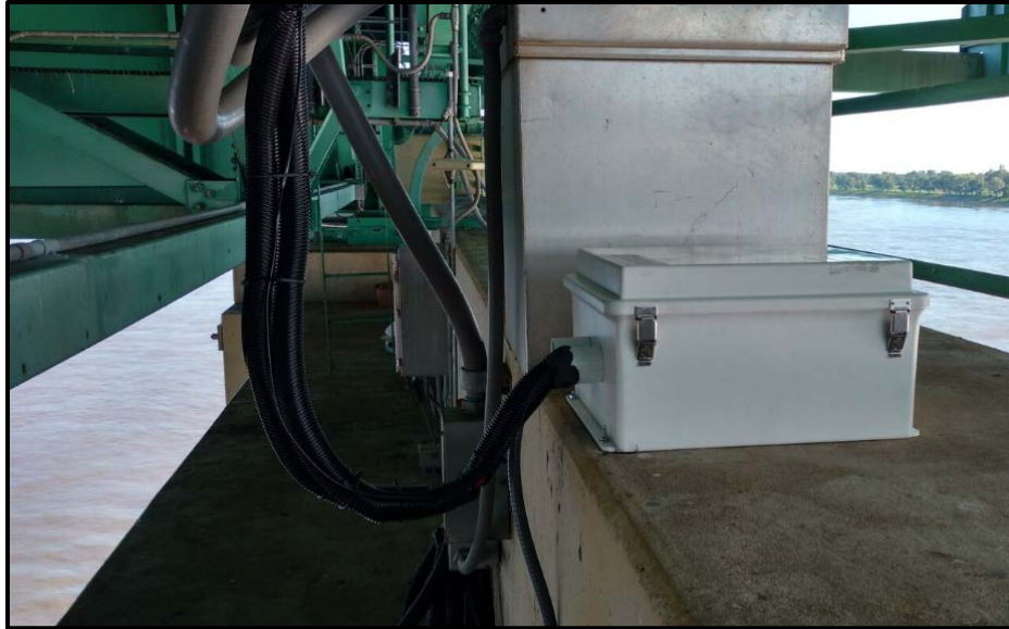
Figure 6.4 - Box A Post Installation
