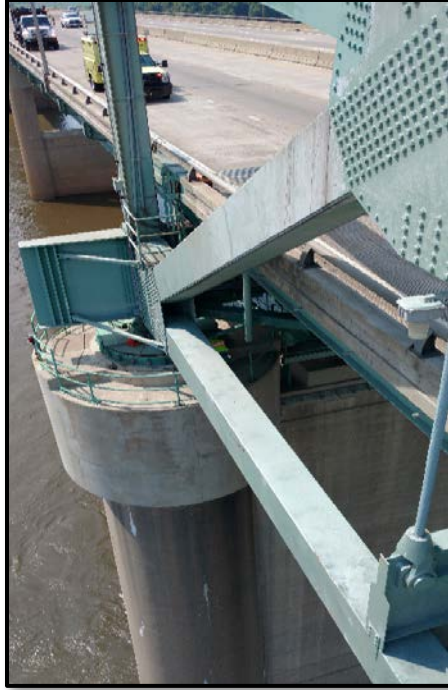
Figure 3.5 – Arch Member Framing into the Bearing
