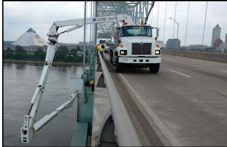
Figure 6.1 - Aspen A-62 Snooper Truck and Road Crew
