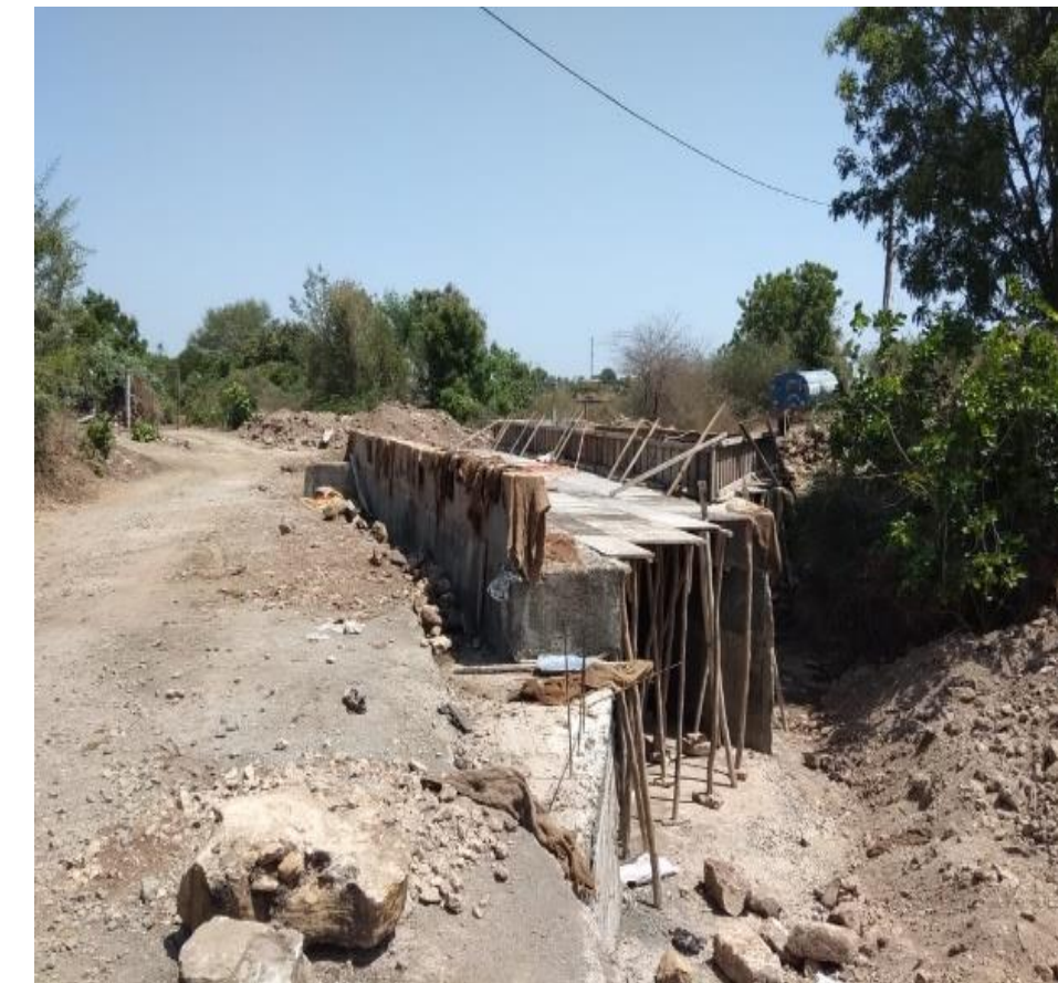
Culverts under construction by Public Works Department
