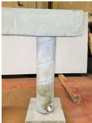
(e) Grout outlet in the column
