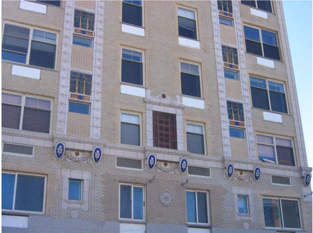
Atlantic Arts Building, 636 Pacific Street
