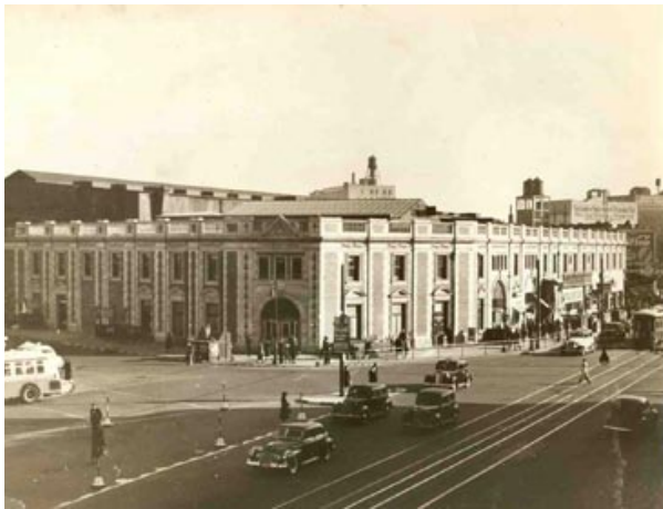
FIGURE 29. Exterior view of Flatbush Avenue Terminal of the Long Island Railroad, date unavailable.
