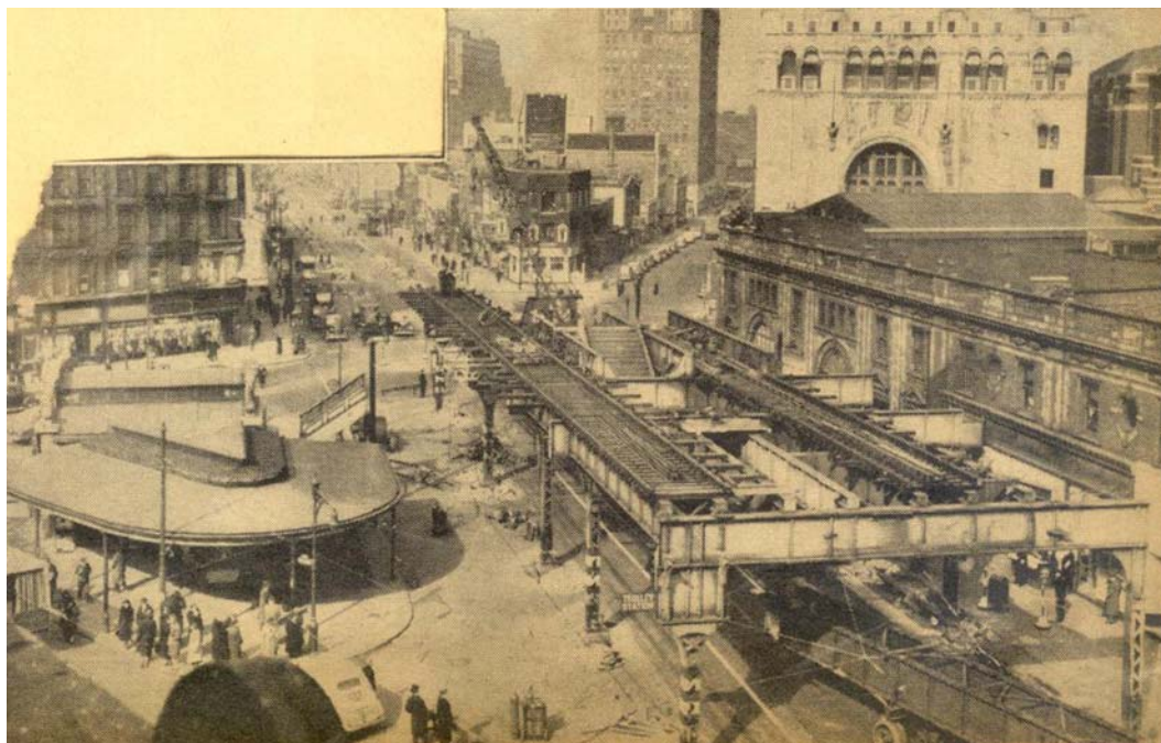
FIGURE 3. Intersection of Flatbush and Atlantic Avenues during El track construction. Middle right, Flatbush Avenue Terminal of the Long Island Railroad; center, El track under construction; middle left, Times Plaza with entrance to LIRR, date unknown.
