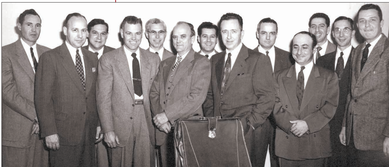
Operations, Construction, and AEC personnel pose in photograph taken in 221-F on December 28, 1954, commemorating the first shipment of plutonium from Savannah River. The photograph was first published in 1972 in the Savannah River Plant News . Its caption identifies the individuals as well as their 1972 job titles. "From left, Julian D. Ellett, general superintendent of Production and now manager of Du Pont Atomic Energy Division; Henry Greene, assistant plant manager; Sam Smiley, Separations; Don Miller, first plant manager; James J. Urban, Separations; Curtis A. Nelson, manager of AEC Savannah River Operations Office; Lowry Danser, Separations; Robert K. Mason, Construction field project manager; James K. Lower, Separations, now assistant plant manager; and Ralph Rosette, Julius Rubin, Goff Giboney and Dave Low, all of SROO." Source: Savannah River Plant News , Vol. XX, No. 1, February 18, 1972. Courtesy of SRS Archives, negative 1511007.
