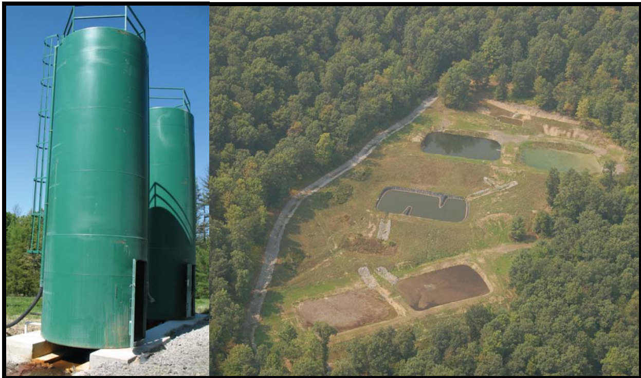
Note: Active system on left shows lime dosers on Porcupine Run in the Bennett Branch watershed. Passive system on right is on Middle Branch in the Kettle Creek watershed. Photo credits: Amy Wolfe.
