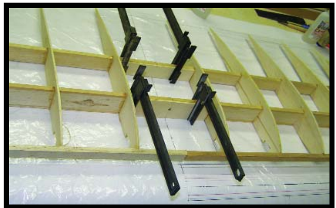
The wing halves are joined with plywood joiners. Notice that the location of the ribs is marked onto the spars.
