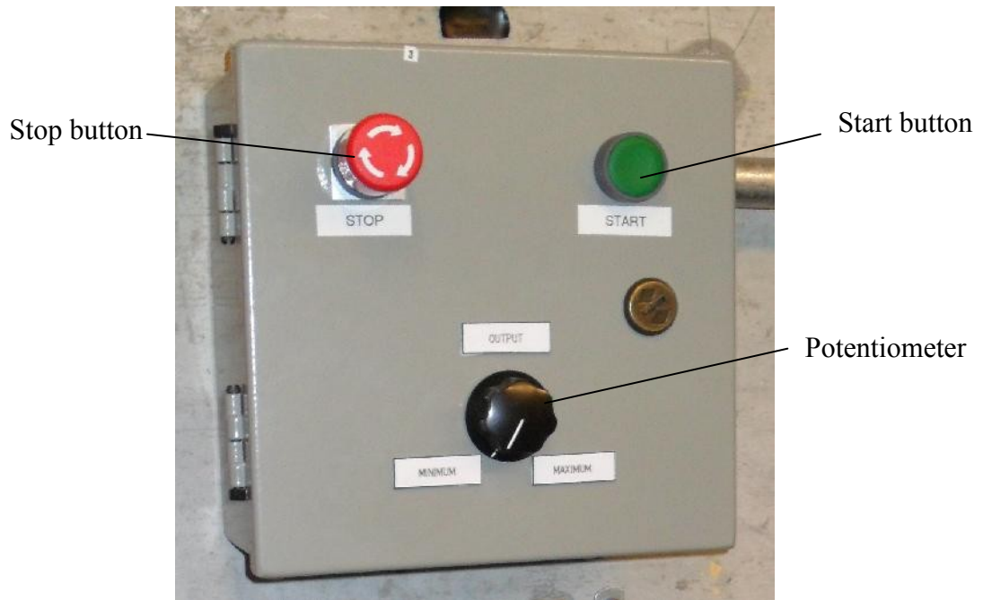
Figure A.22 – Heating power control
