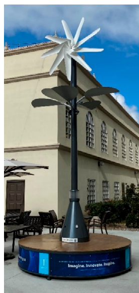
Figure 1. The PrimoWind EnergiPlant, a solar and wind electric charging station installed on our campus.
