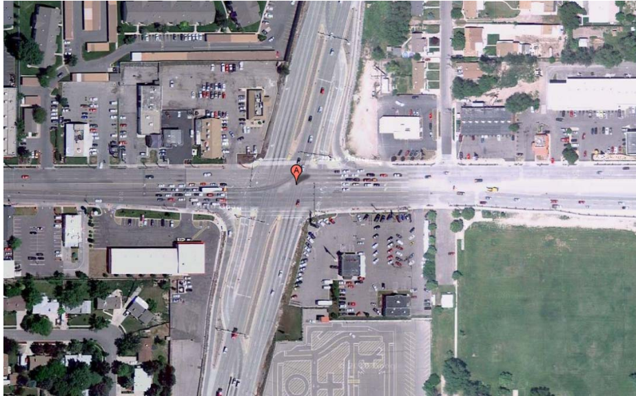
Figure 2-8: Bird's eye view of the CFI between 3500 South and Bangerter Highway in Salt Lake City, UT
